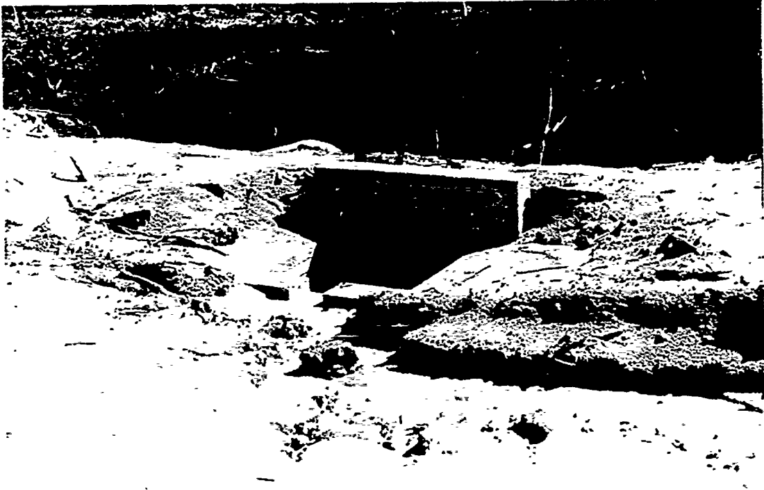
Photo 3-5 Unprotected storm sewer drop inlet on Winslow Way road cut. Sediment flows freely into creek through this.
