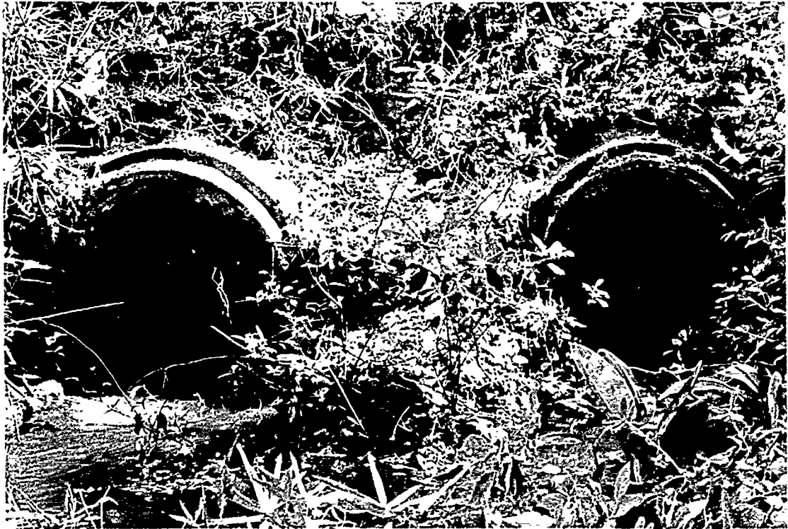
Photo 1-1 Downstream section of 30" and 36" concrete pipes.
