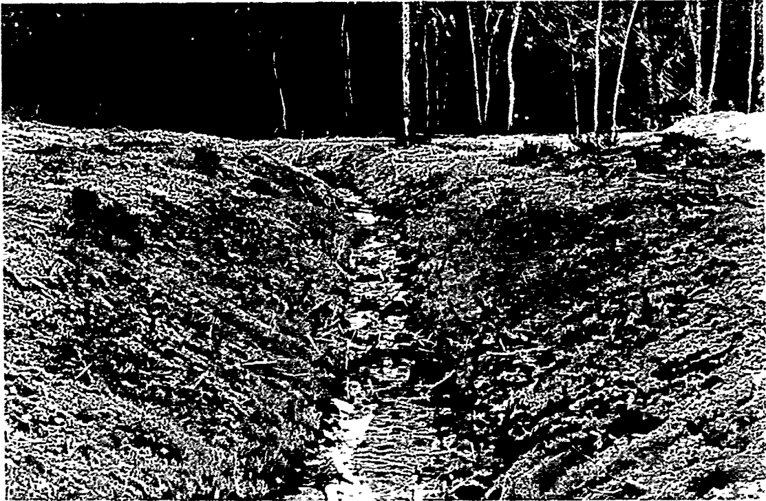
Photo 3-12 View upstream to cross-section #5 on Thornfield Creek. Note growth of grass seed emulsion. August 9, 1990.
