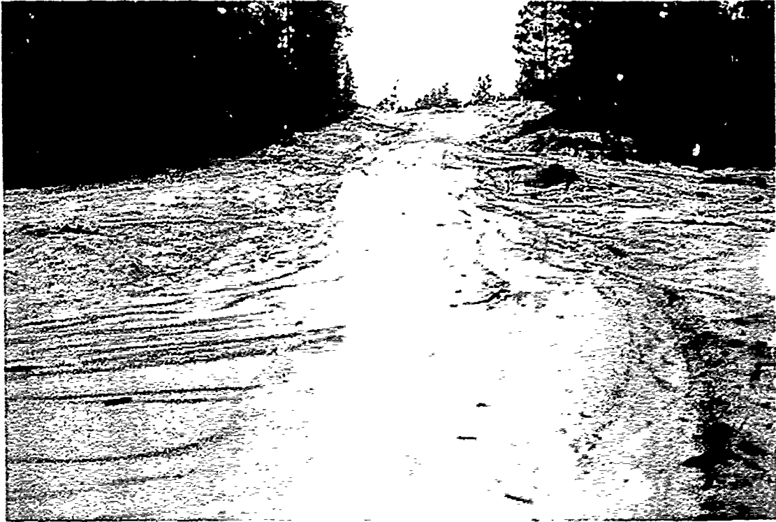
Photo 3-1 View up Winslow Way road cut, October 10, 1990. Sediment is transported directly into channel.
