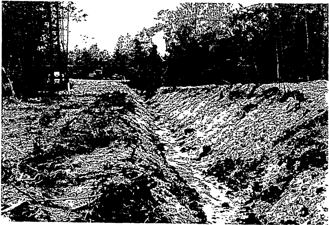
Photo 1-2 Upstream view of Moss Field Creek. Channel improvements include deepening and widening of channel.
