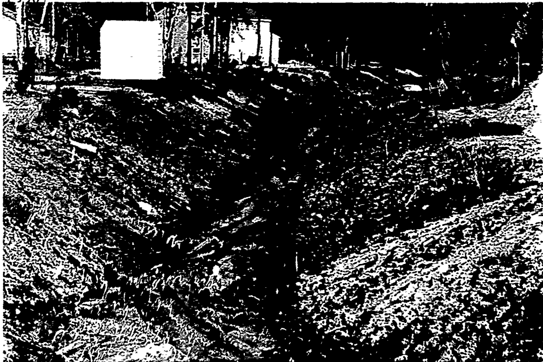
Photo 3-15 View downstream to cross-section #6 on Thornfield Creek near log. Grass at cross-section is stabilizing channel banks. August 31, 1990.
