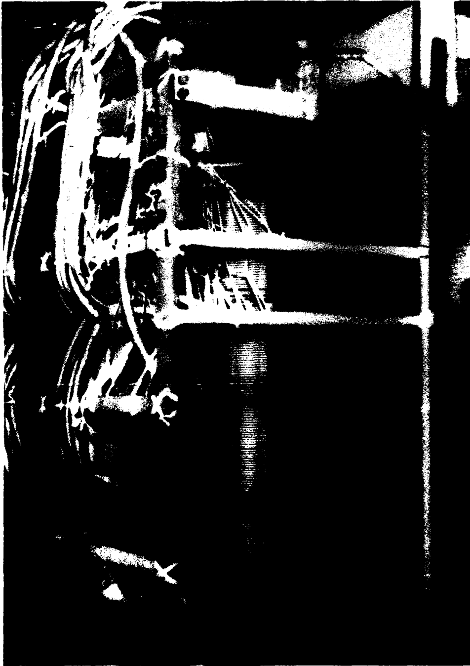
Fig. 2.9. Outboard phase of the 16.4-MVA core-form power transformer with sensing leads and temporary terminal board in place, ready for retanking.
