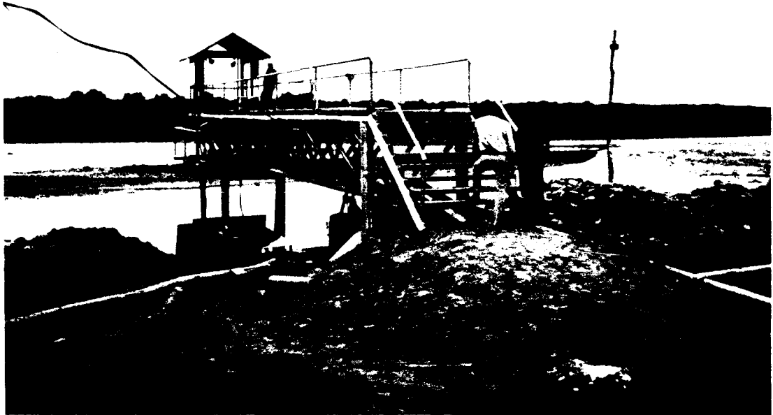
Photo 21. Water Intake Esquema Irrigation Project - Rio Pilcomayo Near Villa Montes
