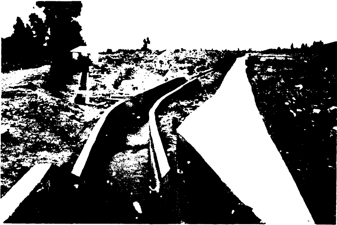
Photo 6. Punata Tiraque Irrigation Project Showing Irrigation System Channels
