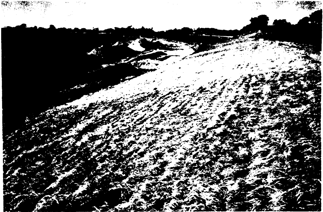
Photo 24. Flood Control Levee Under Construction on Rio Piray - City of Santa Cruz
