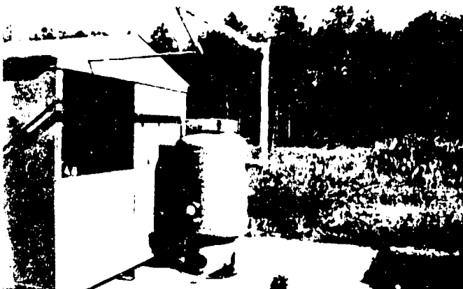
The air is pumped into a pressurized holding tank and delivered through the piping that is marked breathing air. This is a dedicated breathing air system, an excellent practice.
