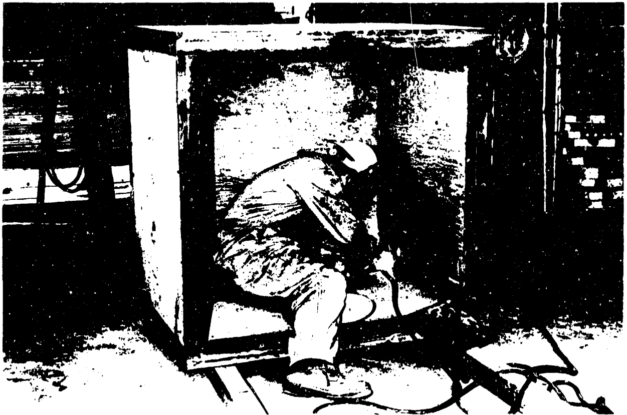
Welding the SIFCON Panels Together Figure 10.
