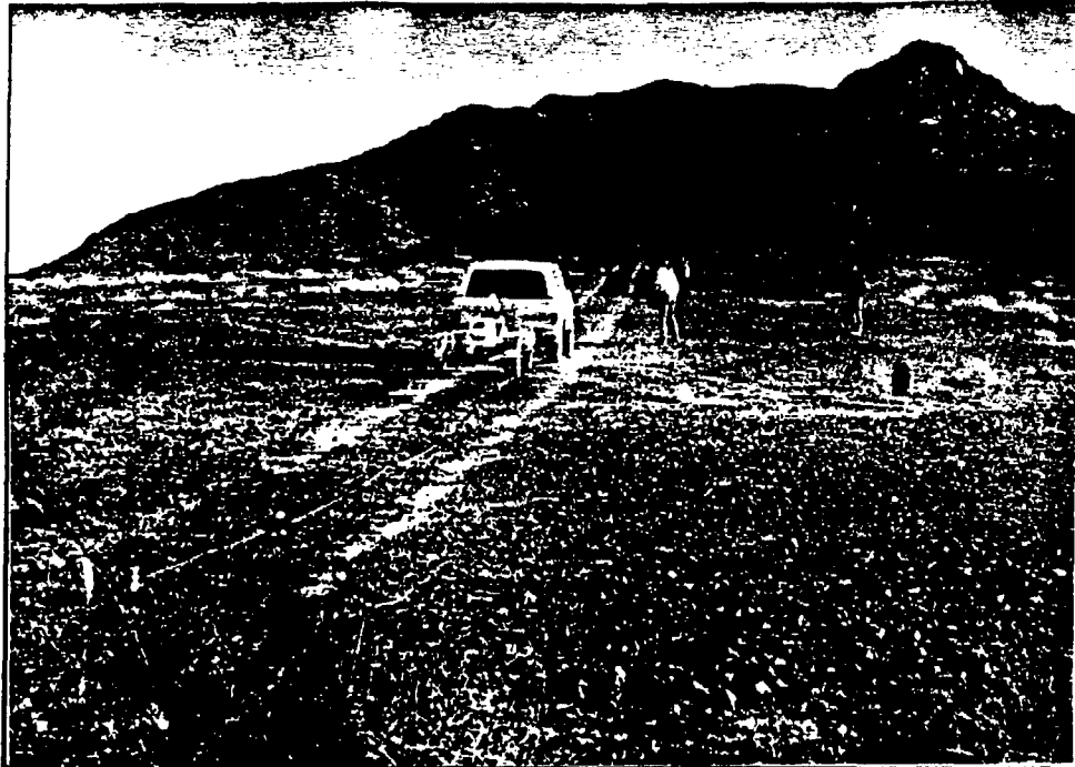
PHOTOGRAPH NO. 2017399-07 APG Profilometer on Middle East Course No. 2 Track Width on APG Profilometer Was 48"
