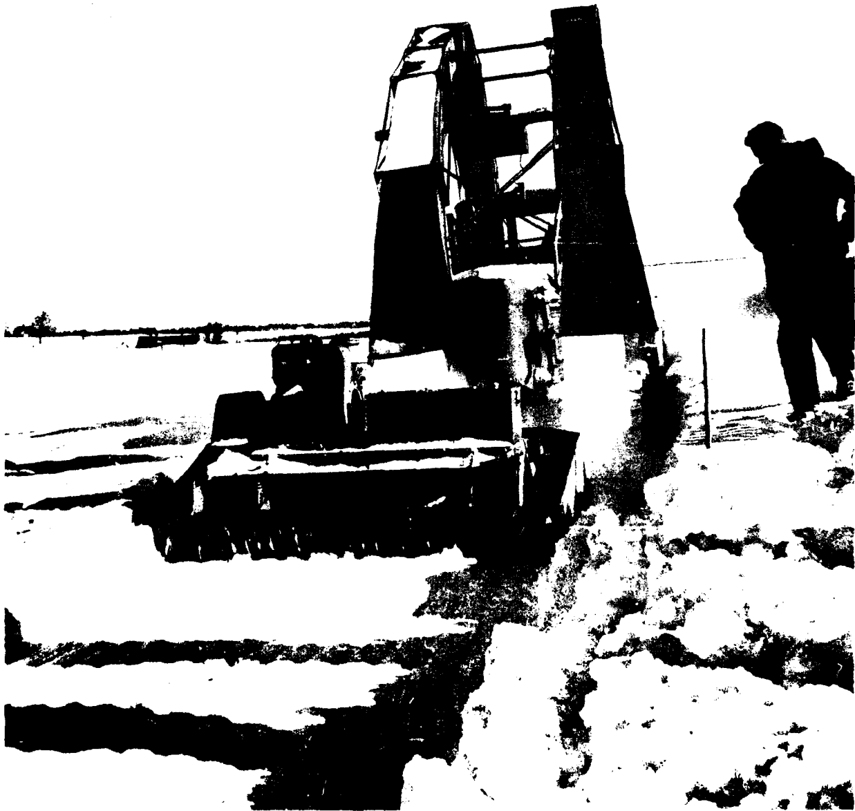
Figure 92. Vibratory compactor towed by Peter miller.
