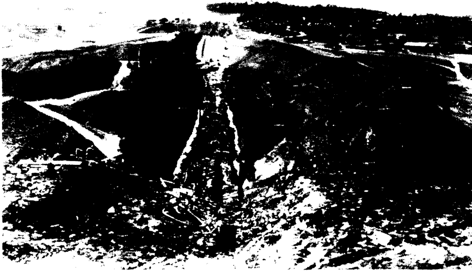
Figure 19. Completed core trench excavation, looking southwest from left abutment to right abutment (FOL-619, 9/26/51)
