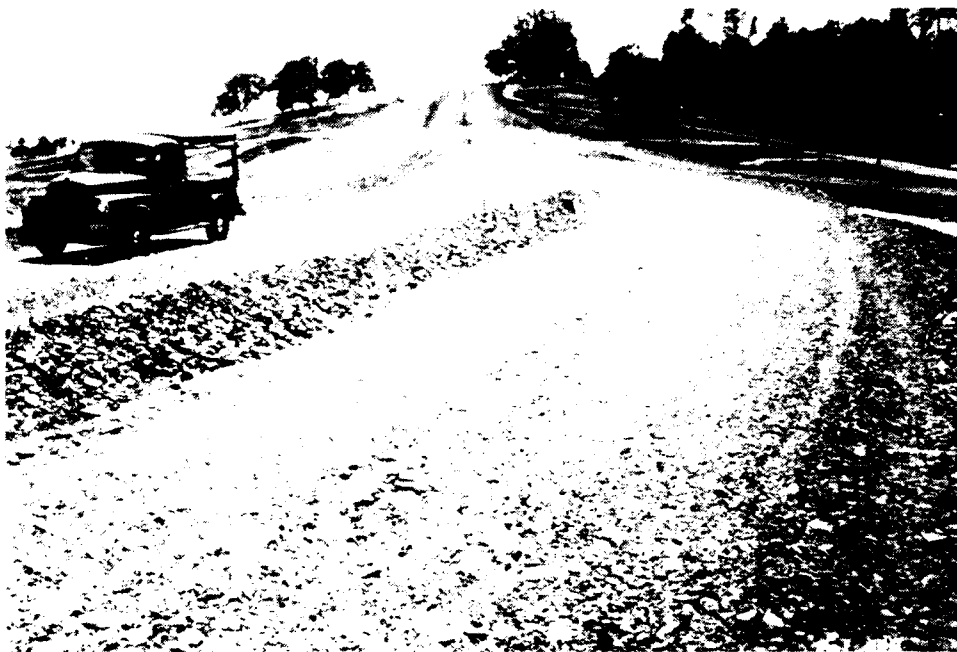
Figure 21. Placement of Zone 1 upstream shell, looking southwest from sta 421+50 to right abutment (FOL-528)
