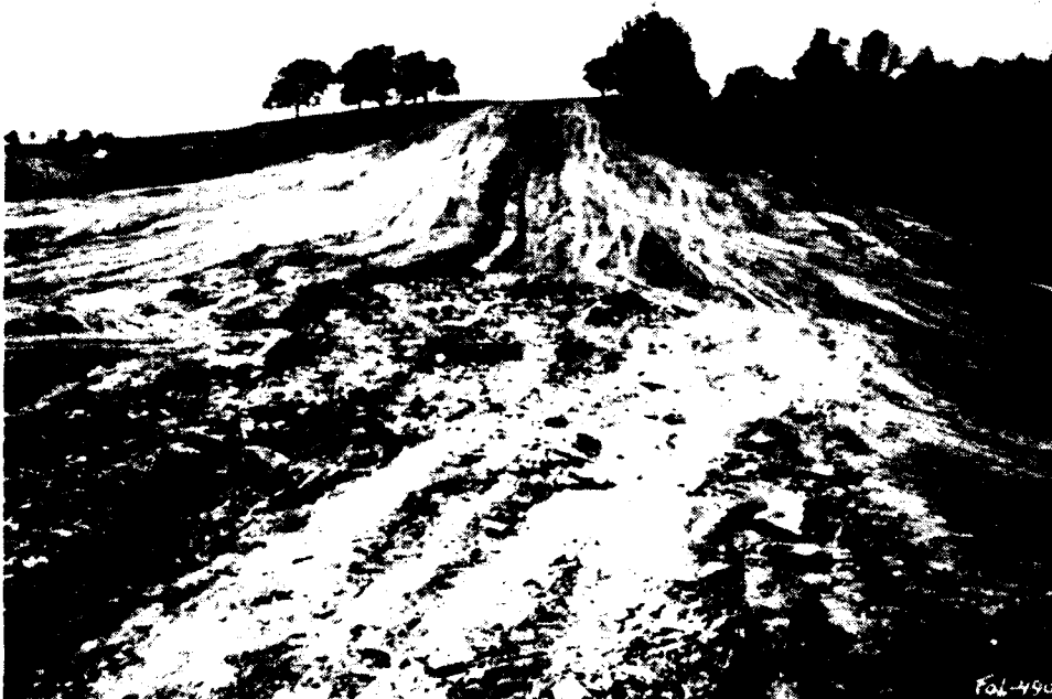
Figure 16. Foundation preparation for portion of Mormon Island Auxiliary Dam founded on rock, looking southwest from sta 421+00 to right abutment (FOL-490, 4/11/51)
