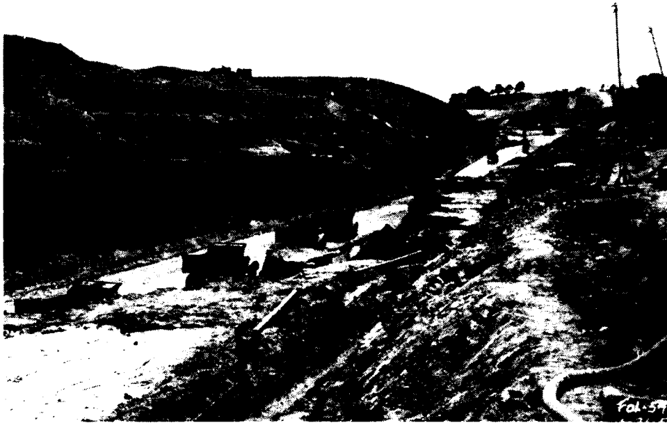
Figure 17. Core trench excavation through undisturbed alluvium, looking southwest from sta 440+00 to right abutment (FOL-544, 6/25/51)
