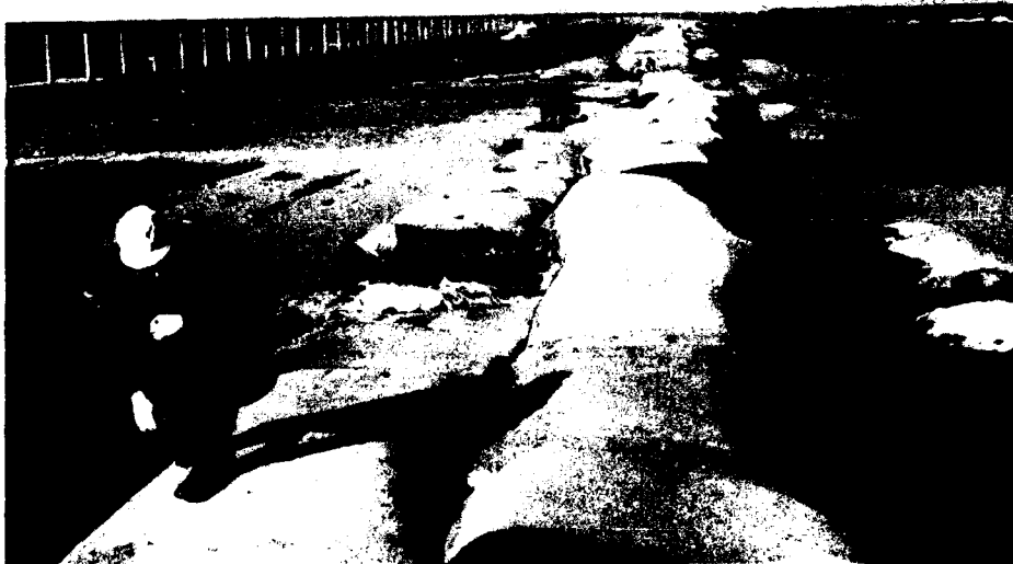
d. Dike after exposure to the elements for 2 years
