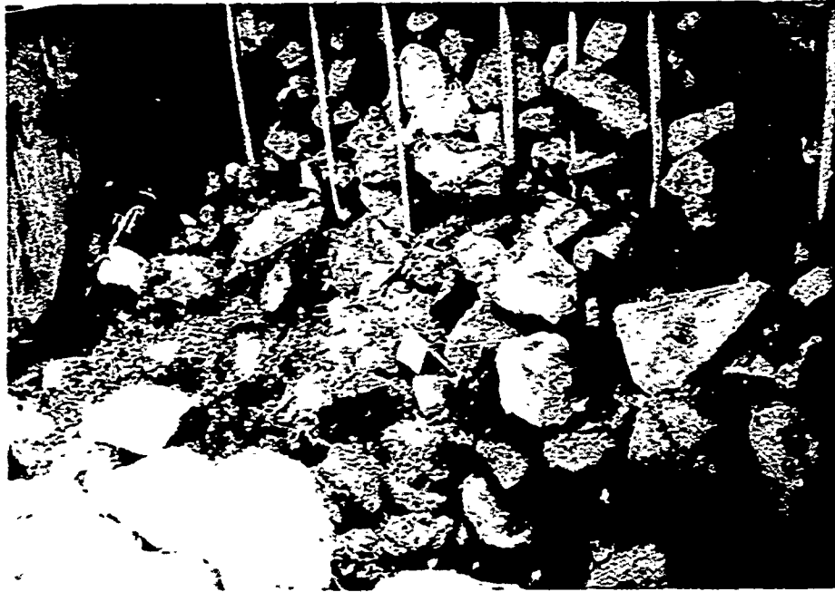
Figure 43. Section C, Phase 2 disassembly. (Sodium Silicate-Cement Mixture of chemical sealant placed by W. G. Jaques Company, Des Moines, IA)
