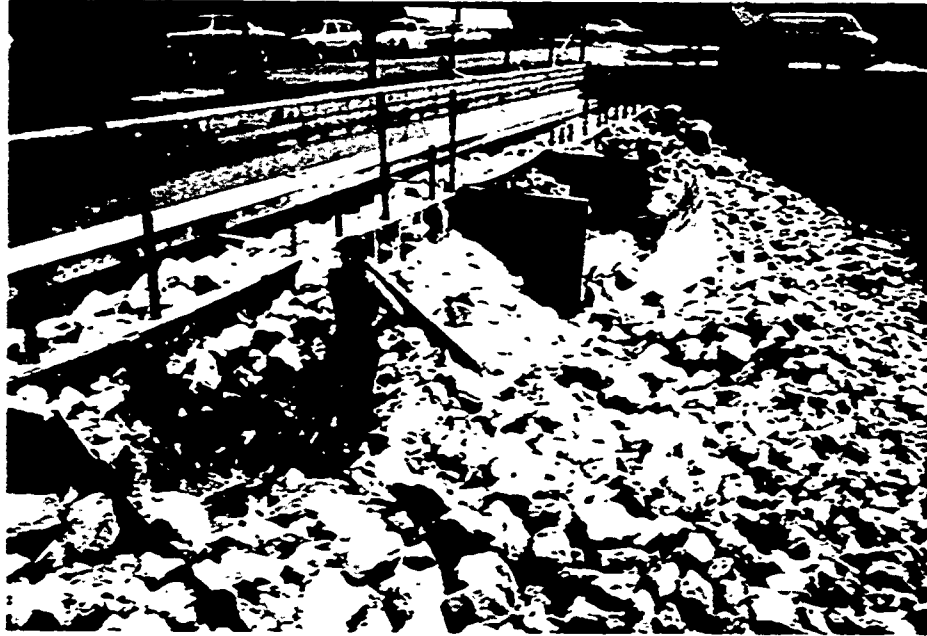
Figure 34. Disassembly of physical model section for evaluation of Sand-Asphaltic Mixture as potential material for void sealing
