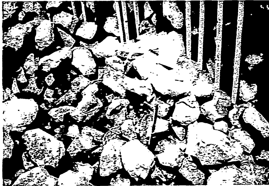
Figure 36. Section A, Phase 1 disassembly. (WES Mixture of cementitious sealant placed by W. G. Jaques Company, Des Moines, IA)
