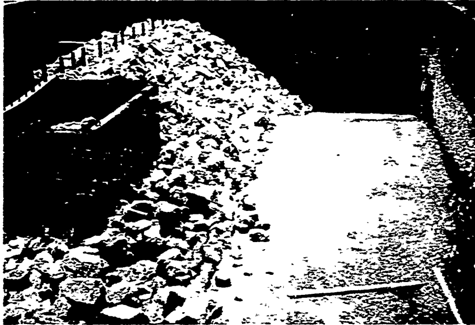
Figure 10. Construction of rubble-mound physical model around saltwater test section to determine salinity effects
