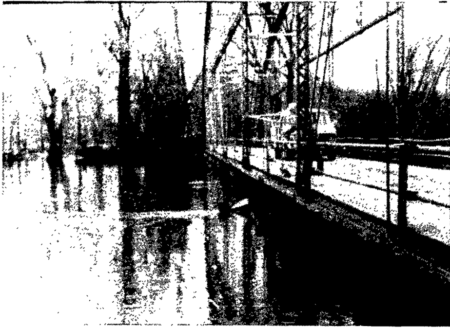
Figure 40. Initiation of sampling with Helley-Smith bed-load sampler
