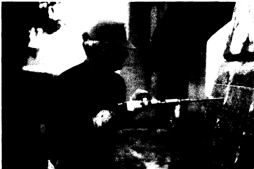
Figure 21. Wet drilling of port holes
