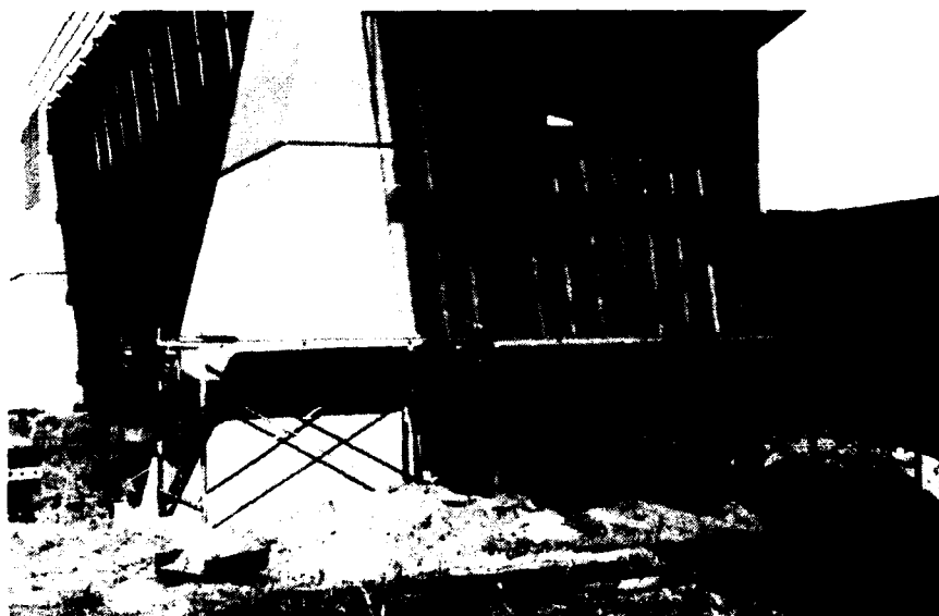
Figure 12. Construction scaffolding in place around pier
