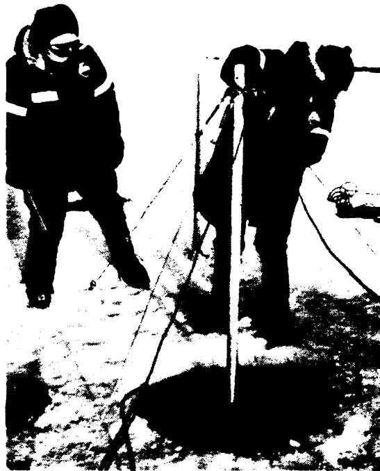
Figure 6. Attaching wires to hold the pole vertical after the block has been pushed down.
