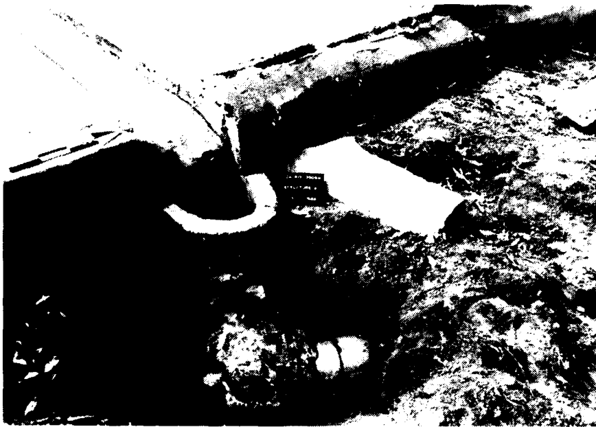
Figure 4.42. Structure 6, Milking Barn, gutter drain; looking northwest.
