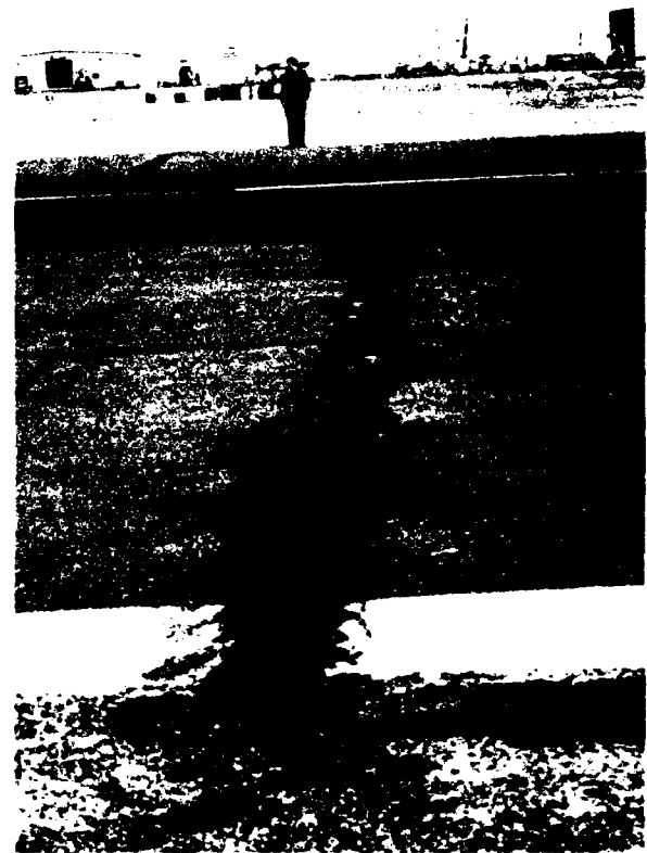
Figure 22. Severe earth-related cracking in runway at Deadhorse (Carpenter and VanDam 1985).
