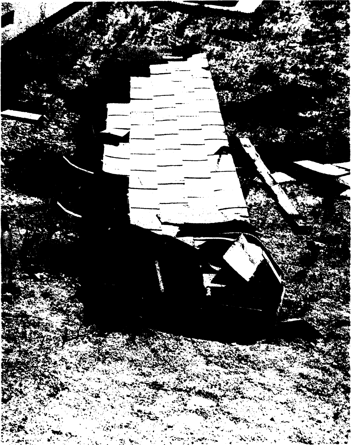
Figure 10. Eave section which fell off a manufactured unit.
