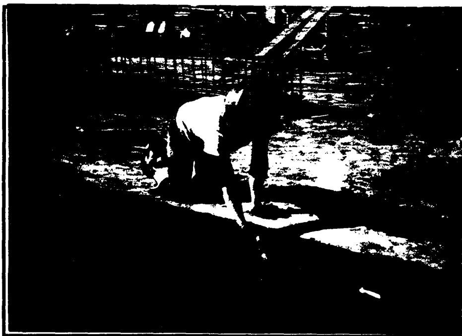
Figure 6.3 Hand Troweling
