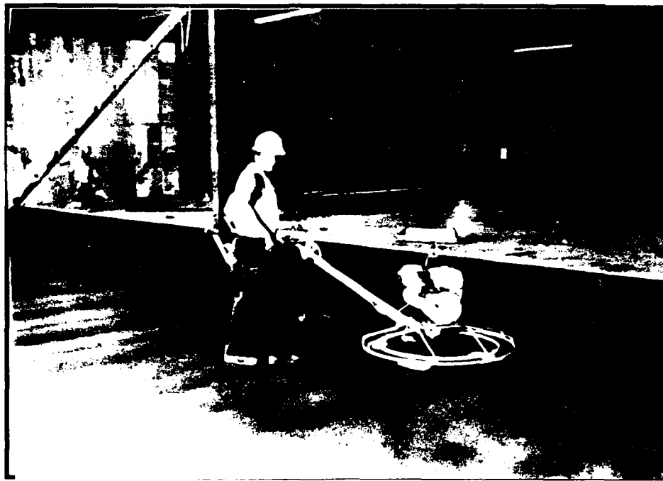
Figure 6.4 Walk-Behind Troweling
