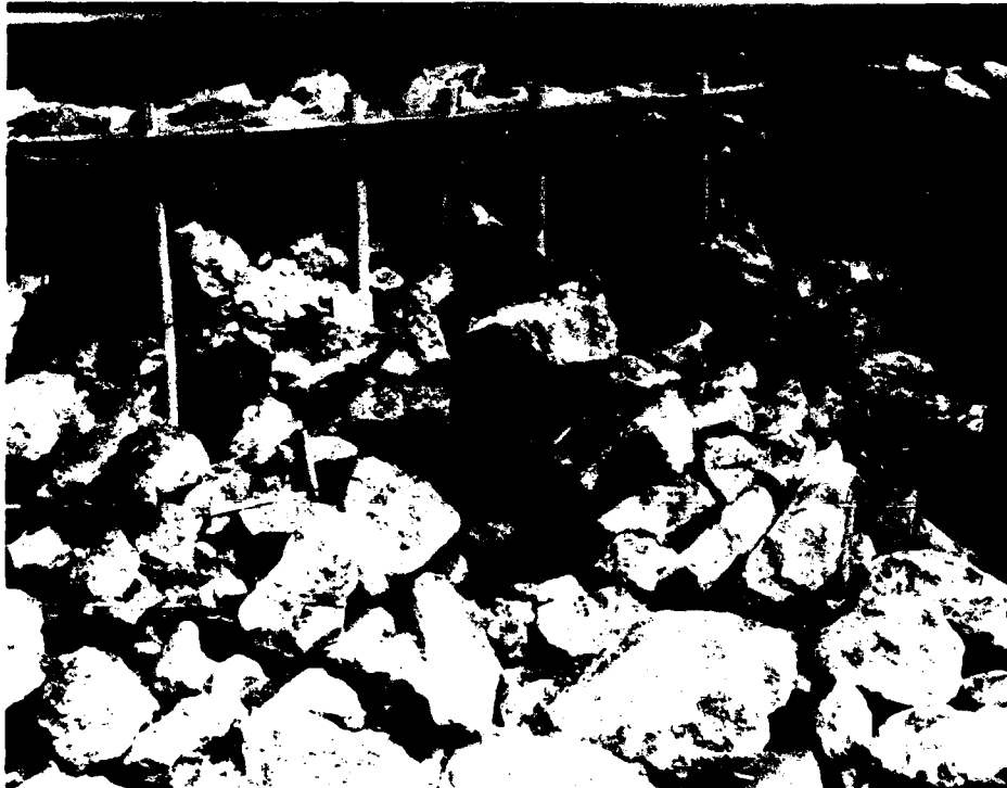
Figure 46. Section C, Phase 1 disassembly of physical model of rubble-mound structure. (Sodium silicate-cement mixture of chemical sealant placed by W. G. Jaques Company, Des Moines, IA)
