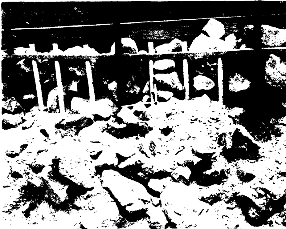
Figure 51. Section D, Phase 1 disassembly of physical model of rubble-mound structure. (Sodium silicate-diacetin mixture for sand stabilization placed by W. G. Jaques Company, Des Moines, IA)
