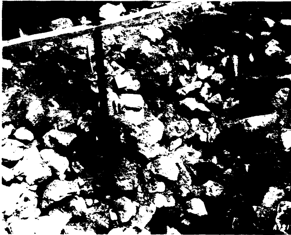
Figure 60. Section E, Phase 2 disassembly of physical model of rubble-mound structure. (Mastic asphalt subjected to irregular splashing caused by temperature differences between mastic and water-filled voids, placed by WES Geotechnical Laboratory personnel)
