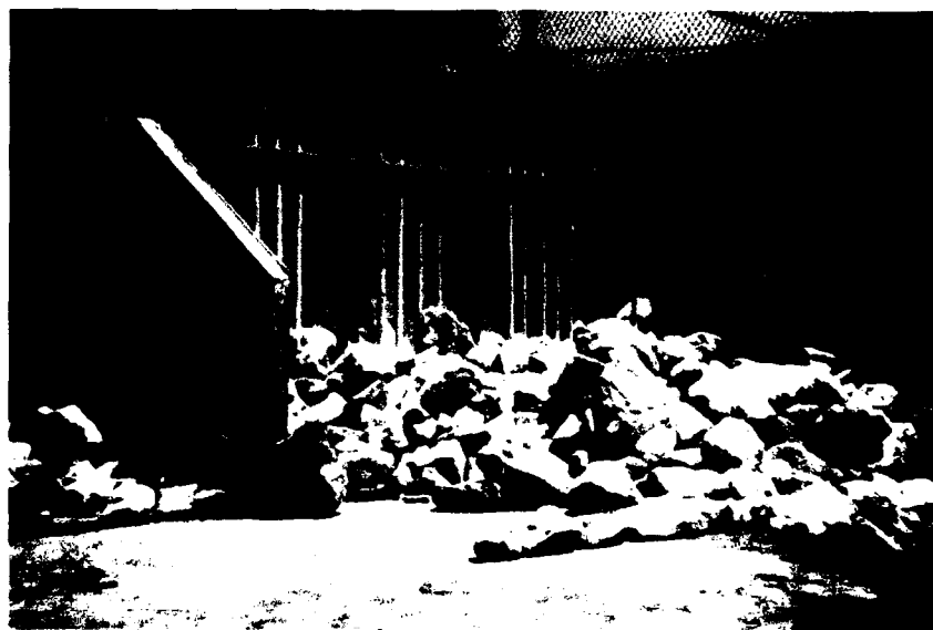
Figure 9. Placing stone around sealant pipes and instrumentation conduits in physical model of rubble-mound breakwater or jetty
