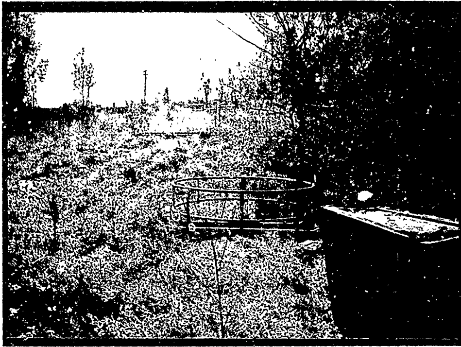
21. SEWAGE TREATMENT PLANT AREA
