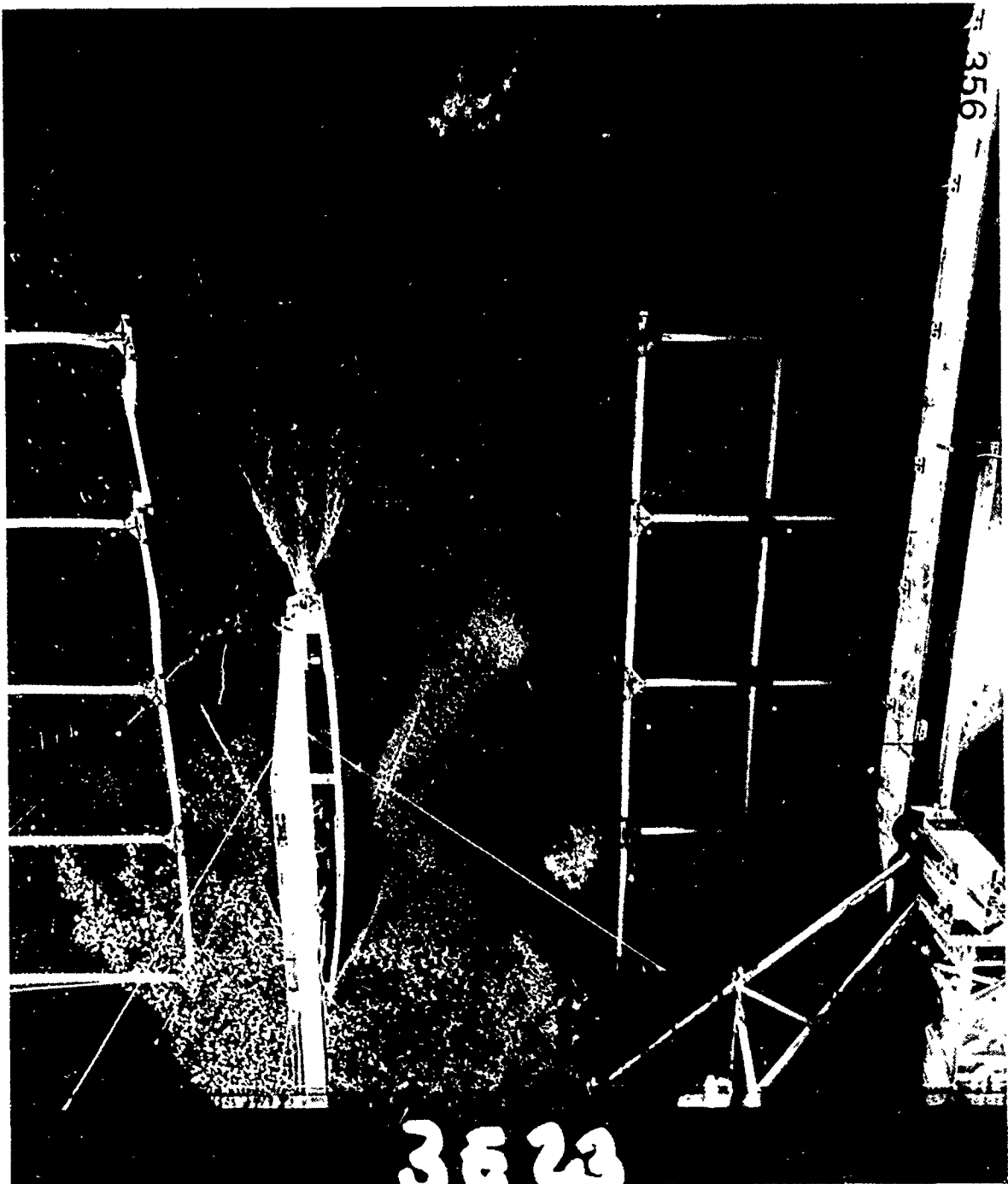
Fig. 48. Photograph of the Kelvin wake generated by Model 4645 at F_n = 0.31 .
