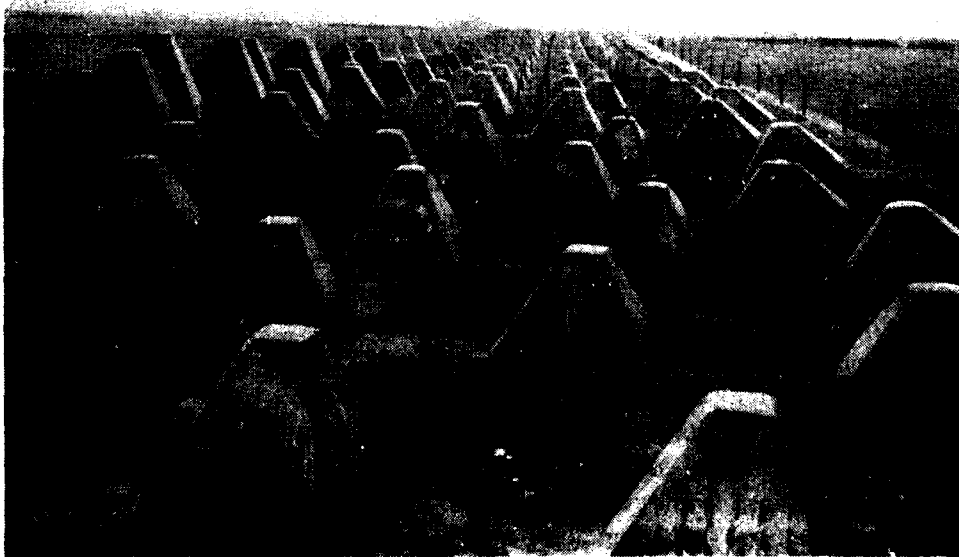
Too obtrusive to construct in West Germany today, but an effective wartime obstacle fifty years ago, these concrete dragon's teeth formed part of the Siegfried Line. This photo was taken near Lammersdorf, Germany, on 25 September 1944.
