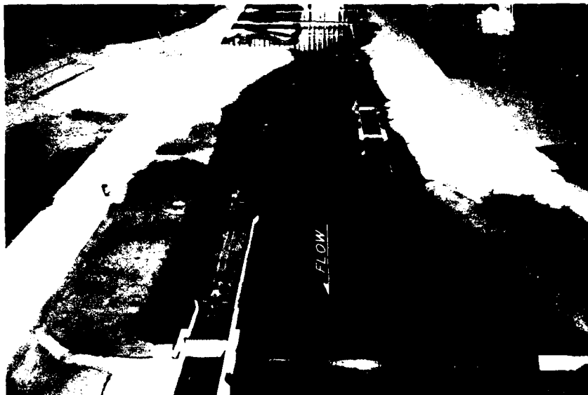
Photo 9. Plan A, looking upstream, discharge 30,000 cfs. Path of upbound tow leaving replacement lock
