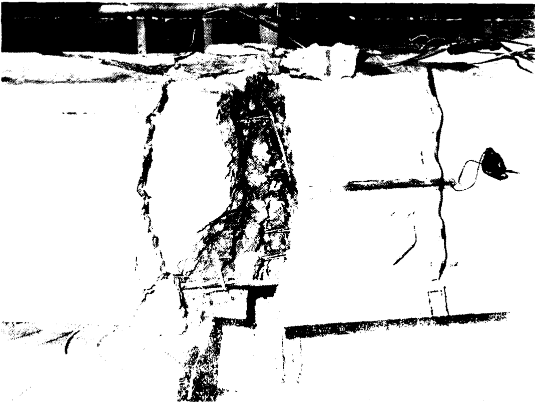
Figure B-168. MK16 compression spalling at failure.
