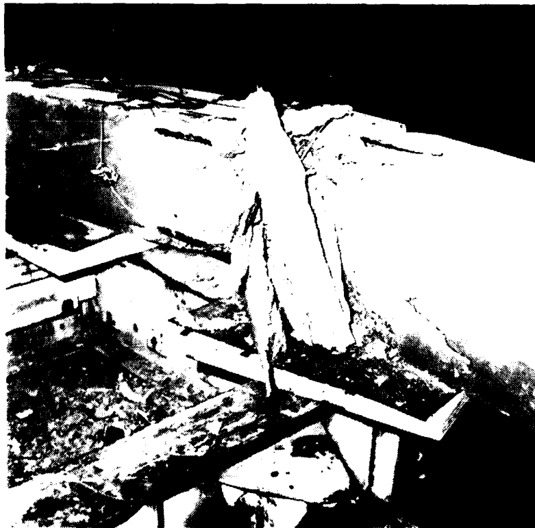
Figure B-264. Compression face after failure of COL01.
