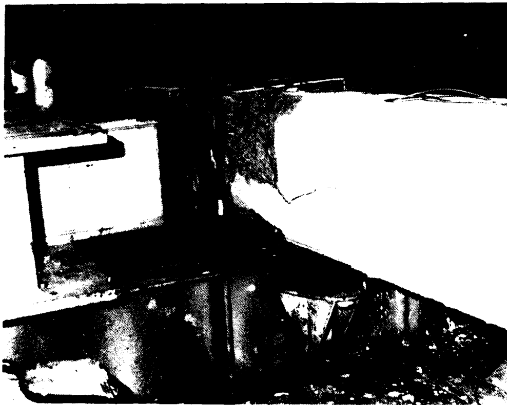
Figure B-91. MK8 ultimate load spalling.
