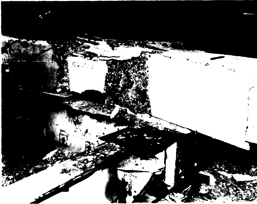
Figure B-277. Compression zone spall of COL03.
