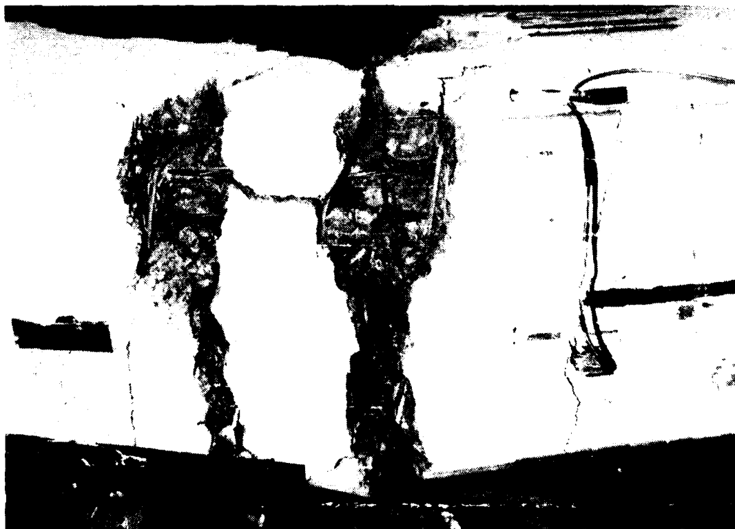
Figure B-207. MK22 tension cracking at failure.
