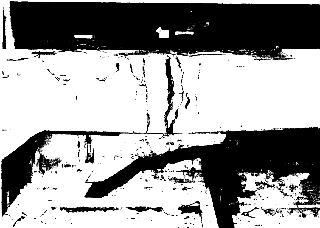
Figure B-232. MK5A tension cracks at failure.
