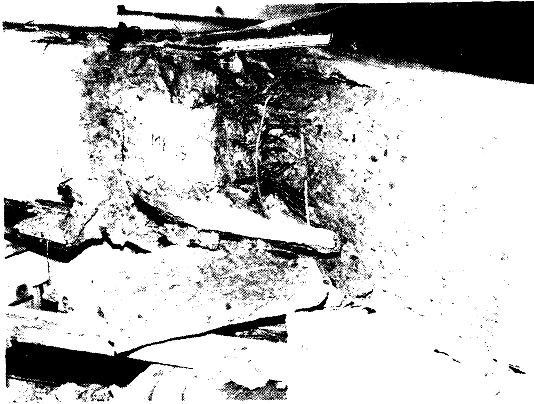
Figure B-187. MK19 compression spalling at failure.
