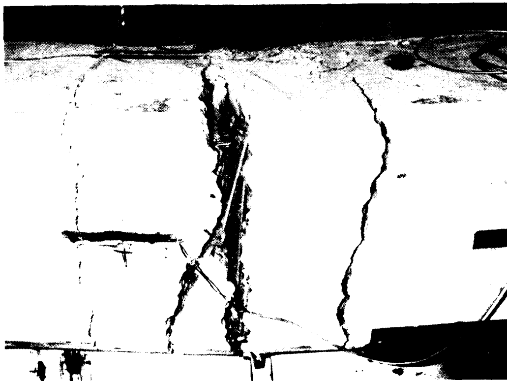
Figure B-216. MK23 tension cracking at failure.
