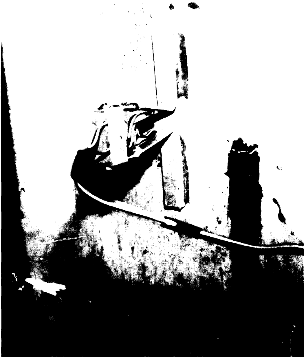
Figure 9. Clip gages for crack width measurements.
