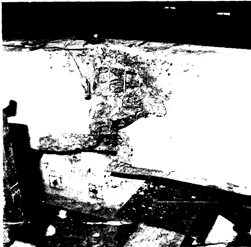
Figure B-146. MK13A compression spalling at failure after monotonic loading.
