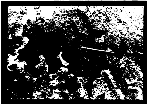
PHOTOS 16 & 17: Separation of top layer of Triple Bituminous Surface Treatment (TBST). May be caused from fuel spills, jet blast, or turning aircraft.
