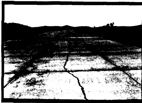
PHOTO 7: Sealed longitudinal crack on Feature T02A.
