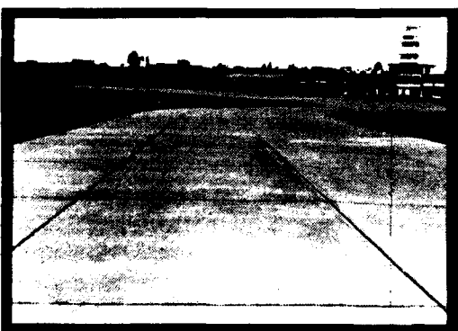
PHOTO 5: Excellent condition PCC typical of many pavements throughout the airfield.
