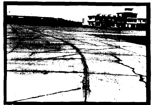
PHOTO 8: Load related cracks that have been well maintained. Traffic is concentrated in this area.
