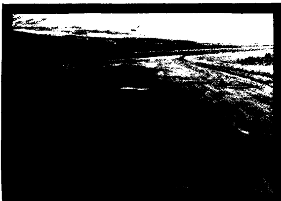
FIGURE 11: Apron access taxiway from the runway. Apron is constructed of Single Bituminous Surface Treatment on a 1" gravel cover of a cement stabilized base course.
