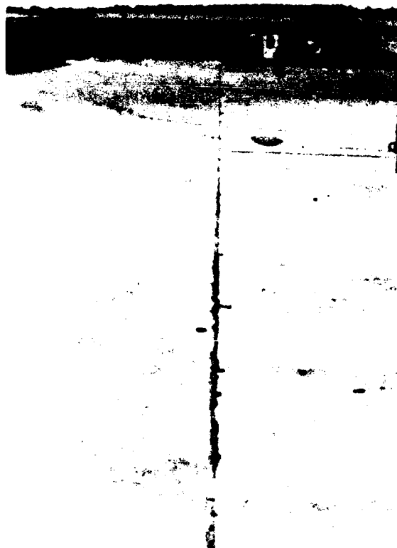
Photo 65. The cold joints were overfilled with joint sealer, causing extrusion of the sealer in hot weather and tearing of the sealer under tank traffic
