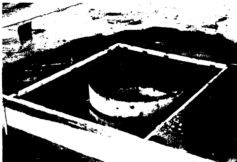
Photo 51. The plate was removed, the manhole built up to the pavement surface, and expansion material used to line the hole
