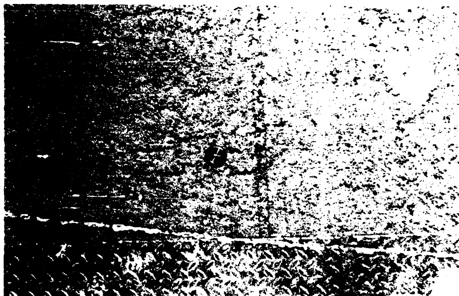
Photo 30. Superficial surface tears parallel to the screed were typical behind the high-density screed, particularly behind the screed extensions (left half of photograph)
