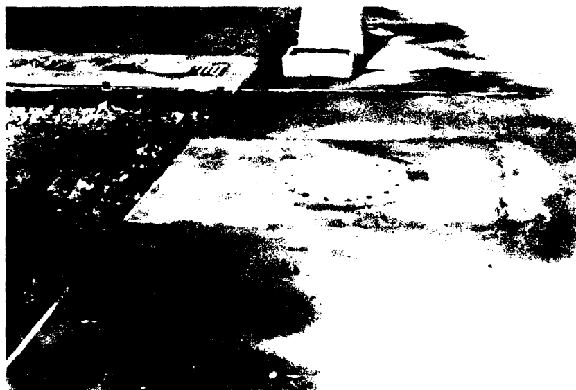
Photo 52. The hole was then filled with conventional concrete to form the finished manhole
