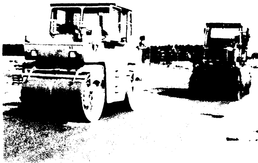
Photo 35. After six or more vibratory passes, the rubber-tire roller made six or more passes to tighten the surface texture
