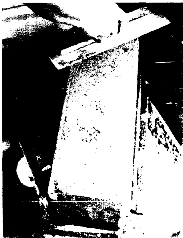
Photo 4. After vibrating the second layer, the beam was finished with a trowel
