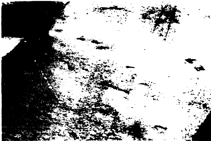
Photo 57. When the RCC was too wet for rolling, roller marks and even footprints were difficult to remove from the surface
