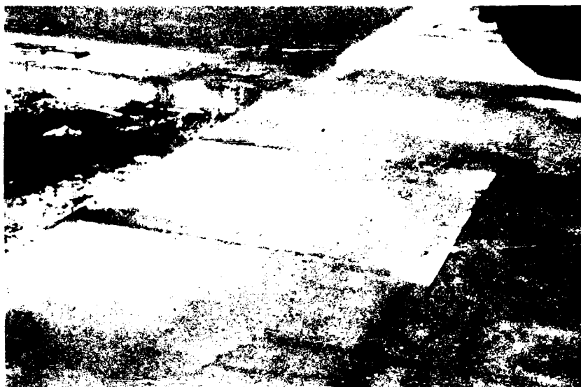
Photo 49. The plate was paved over, and the next day a block of RCC was sawed over the plate
