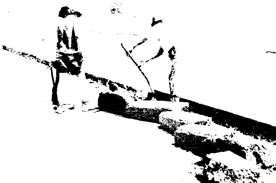
Photo 20. The outer 6 inches to 1 foot along the longitudinal edge was also trimmed with a saw before the adjacent lane was placed
