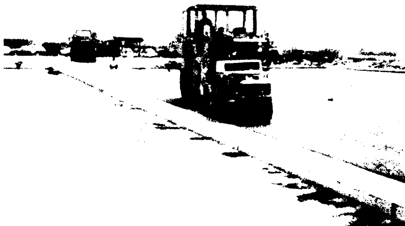
Photo 41. The small vibratory roller was used against the curbs and gutters to protect the conventional concrete from damage caused by the large roller
