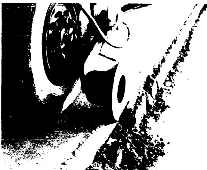
Photo 21. An asphalt cutting wheel was tried for trimming the edge, but it produced an unacceptable joint
