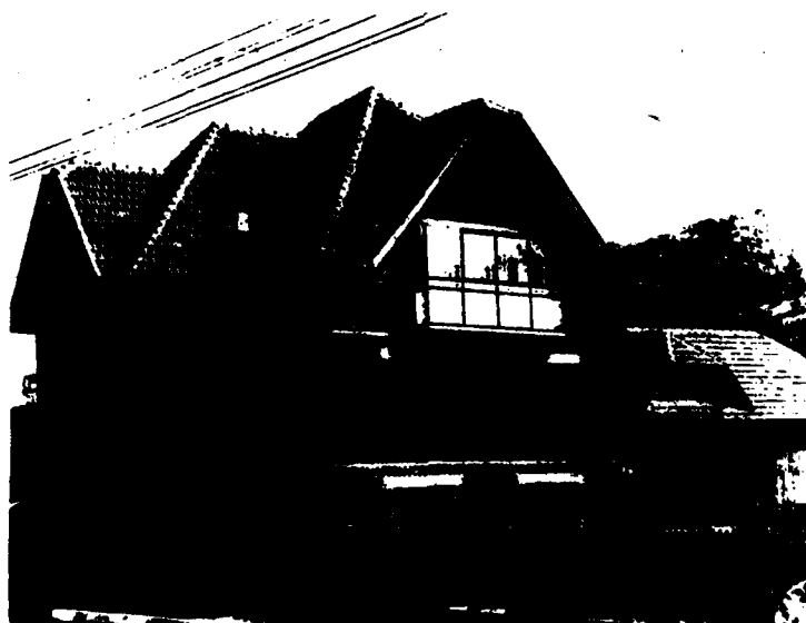
Fig.6. Contemporary rural building before finishing works. Walls:kiln brick masonry.R.C. slabs and lintels. Stone foundation.3 stories. Materials and workmanship quality: very good.Seismic zone:VIII degrees MSK.
