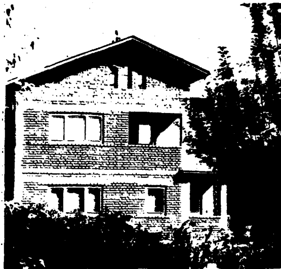
Fig.13. Contemporary, nonengineered rural two storied brick masonry building with embeded r.c. columns and r.c. slabs. Note the tendency to use the collar beam as a frame beam with positive effects on the earthquake behaviour (Seismic zoning in 7th degree MSK).
