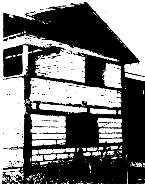
Fig.12. Nonengineered contemporary rural hous- in yitong blocks and reinforced concrete members. Note the r.c. window beam lintel parallel
