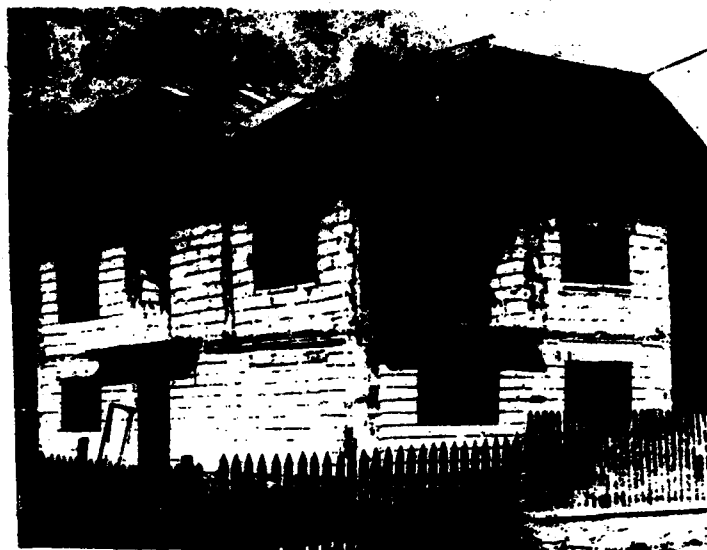
Fig.5. - Contemporary rural building before finishing works. Walls:ytong blocks framed by cast in place r.c. columns lintels and slabs. Stone foundation.3 stories.Upper story in timber.Seismic zone:VIII degrees MSK.Stone and timber available in the region.Materials and workmanship quality: medium.
