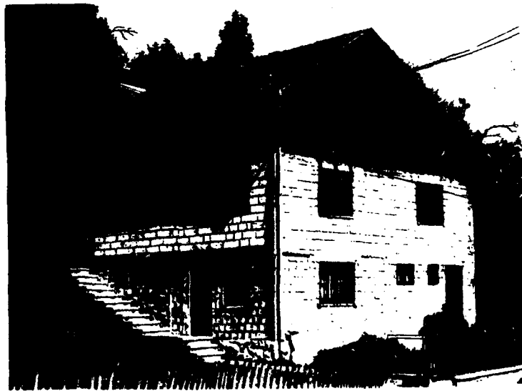
Fig.8. Contemporary rural building: before finishing works. Walls:concrete hollow blocks (1 st. story), ytong blocks (2nd story) and timber (3rd story). Masonry framed by cast in place r.c. columns, collar beams-lintels, slabs. Stone foundation.Seismic zone: VIII degrees MSK. Materials and workmanship quality:very good.
