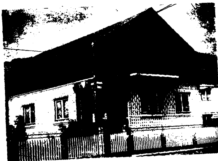
Fig.10. Contemporary rural building after finishing works. First story in masonry, second story in timber. Seismic zone: VIII degrees MSK.
