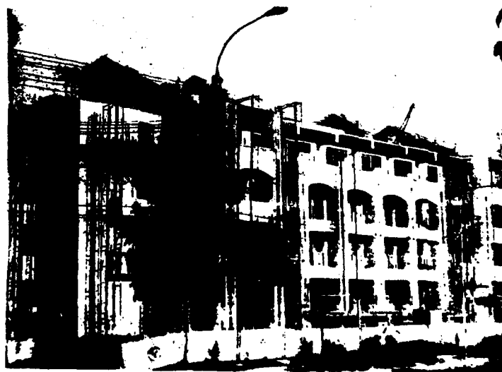
Fig.14. Four storied standard buildings for rural zones using precast members, erected by a specialized construction company near a city. Seismic zone:VII degrees MSK.
