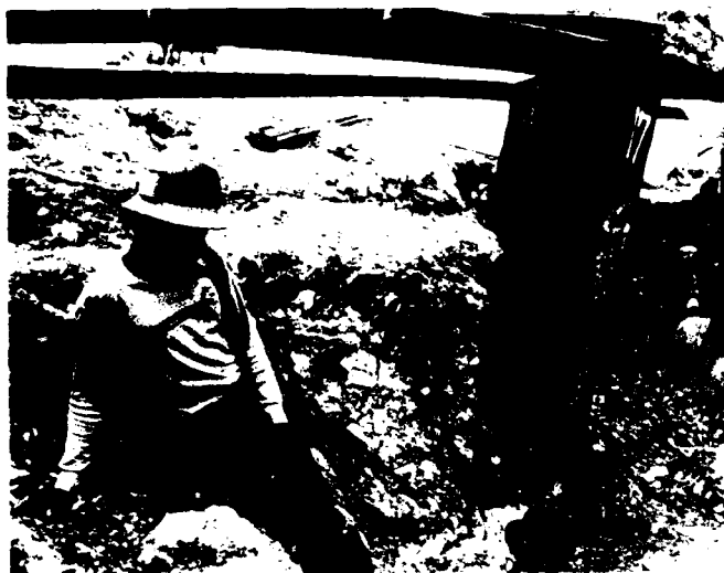
Fig. 13a H-Pile Tilted 18 Deg from Vertical and Heave of Claystone on Slope from the October 1982 Slide
