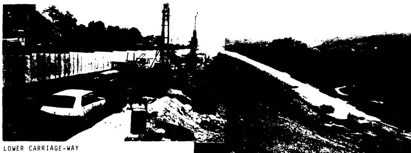
Fig. 6.6 - Plit-levelling of carriage-ways by precast retaining wall and placing of inclinometer tubes to observe the constructed embankment behaviour
