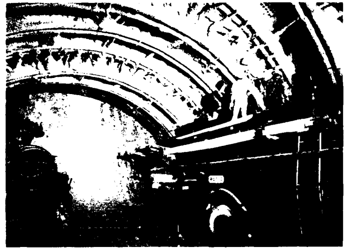
Photograph 2 Drilling for installation of inflaggs (seen stored on drilling rig). Earlier phases of inflaggs ribbing and shot creting seen above the rig. Lumina Motorway Tunnel, Mammola, Italy.
