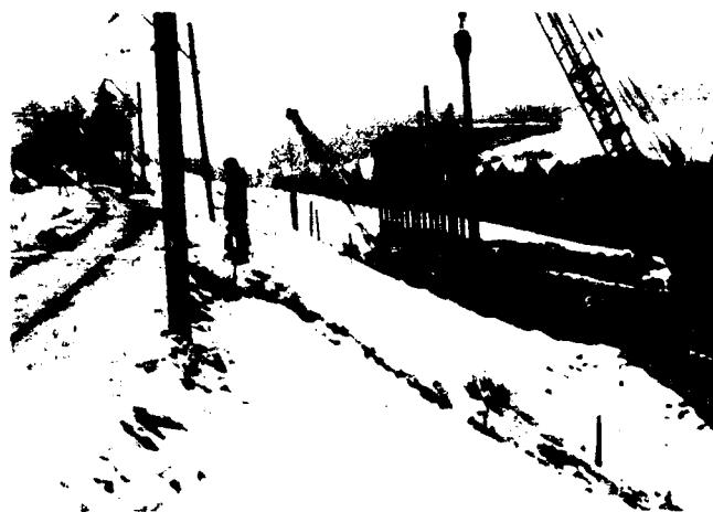
Fig. 2.1 - Railway embankment during Nailing
