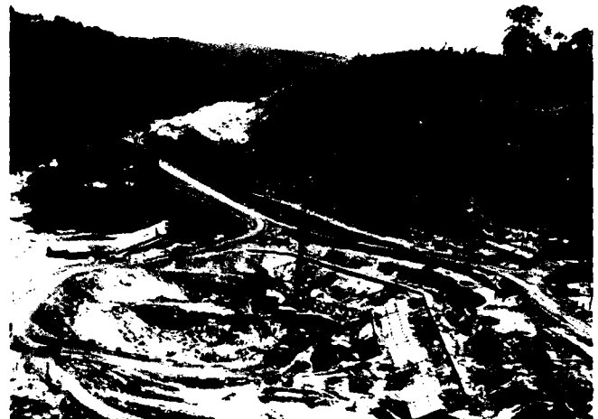
Fig. 3 The Powerhouse Excavation Looking Northwest with the Limestone Ridge in the Background, January 1983, with the Anchored Concrete Restraining System under Construction
