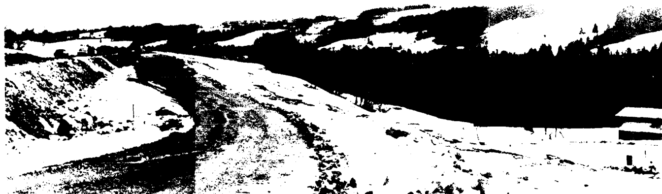
Fig. 6.5 - Second consolidation phase (8 m of embankment) during winter
