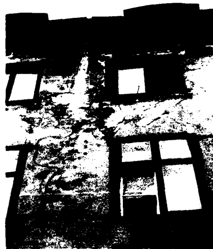
Fig. 5. Cracks in the western façade of House 19 caused by settlements due to piling.
