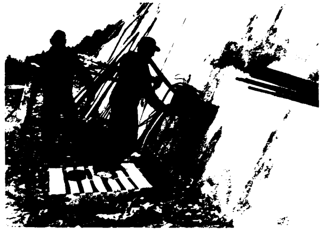
Fig. 5.4 - Tensioning of tie-rods on first anchored slab
