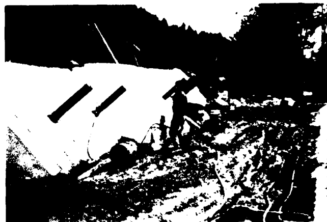
Fig. 4.3 - Execution of 1000 kN anchor-rods
