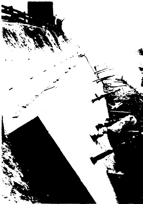
Fig. 5.3 - View of soil nailing and first anchored slab below main Road
