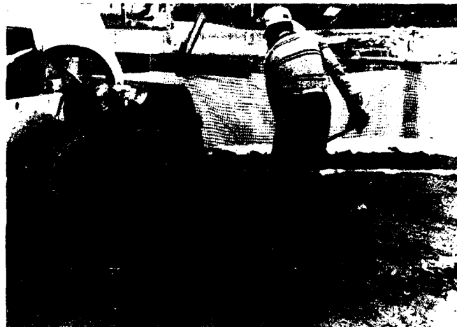
Figure 5. Tensioning of Upper Facing Wrap
