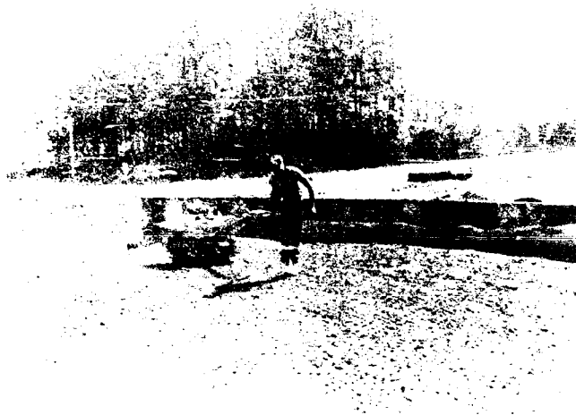
Figure 4. Compaction of Wall Backfill
