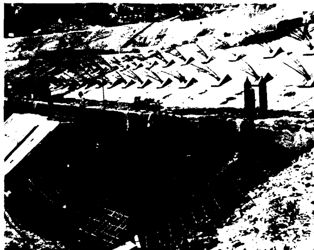
Fig. 16 Constructing the Anchor Concrete Facing Walls to Support the East Excavation Slopes
