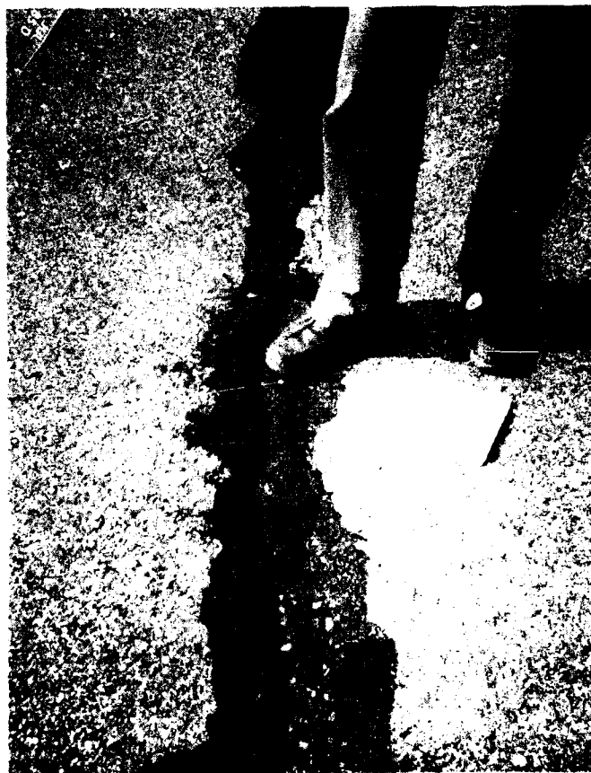
b. Sealant loss into crack.
