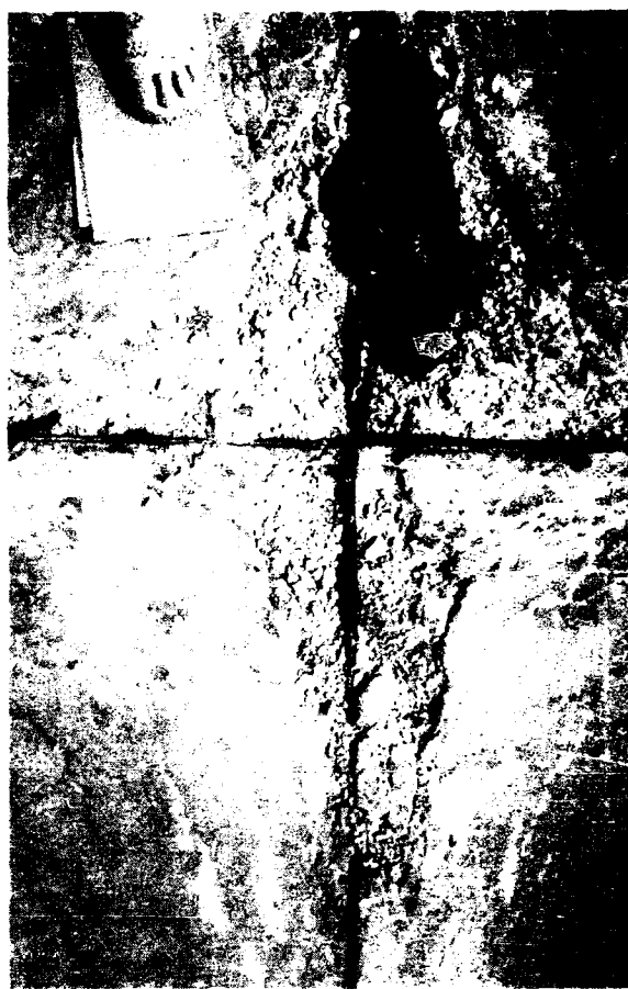
Figure 42. Disintegration in the vicinity of the corner of a PCC pavement.
