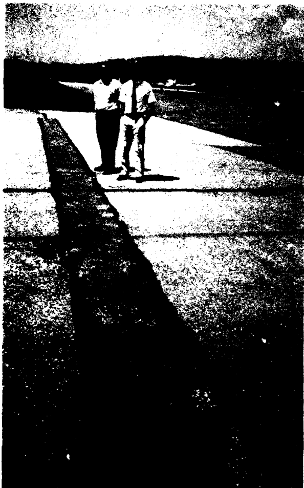
Figure 50. Replaced pavement section to repair multiple transverse crack.
