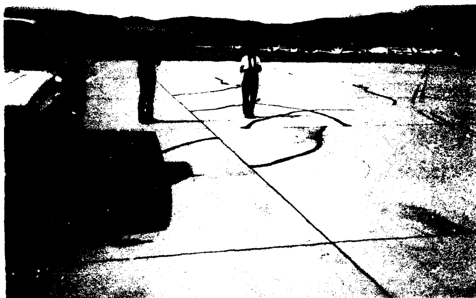
Figure 31. Corner breaks associated with loss of slab support and applied load.
