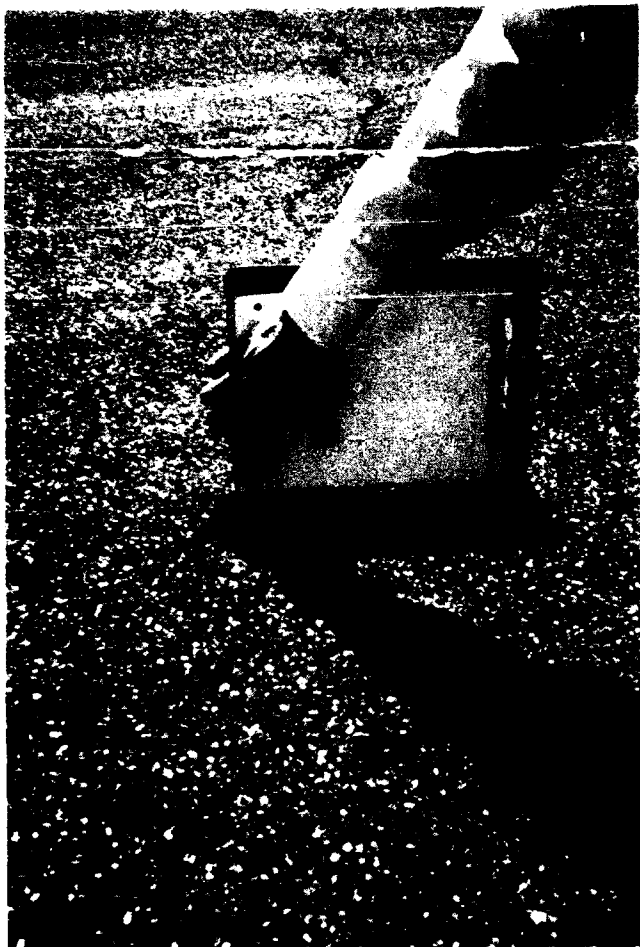
a. "Lipping" at a crack.
