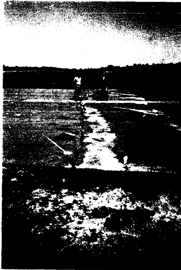
Figure 38. Damage caused by differential frost heave across a backfilled culvert trench.
