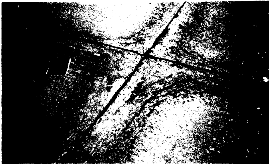
a. Characteristic pattern of "D" cracking in the vicinity of slab corners.
