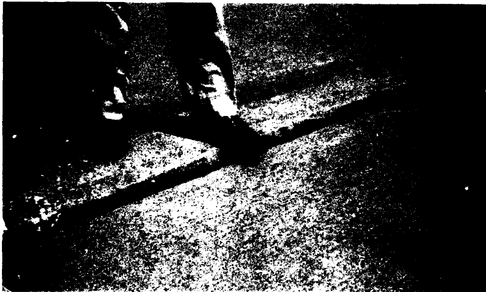
Figure 33. Distortion of PCC pavement surface caused by frost heave.
