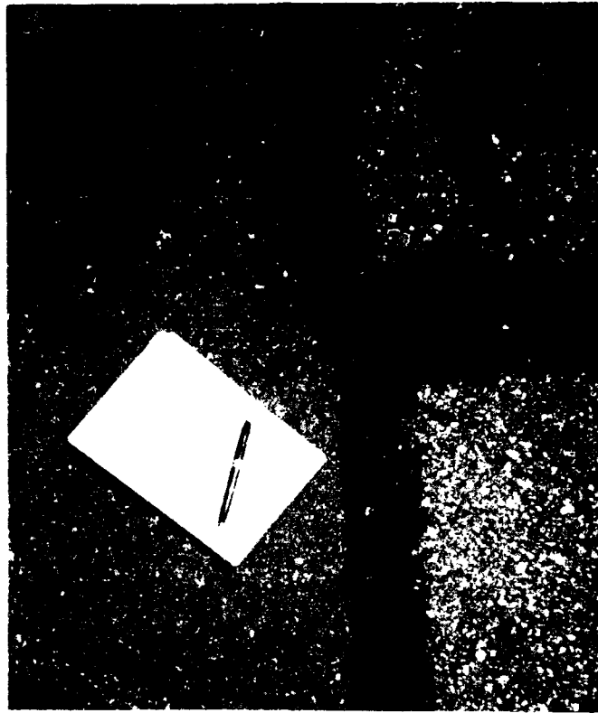
a. Crack at construction joint between replaced pavement section and old pavement structure.
