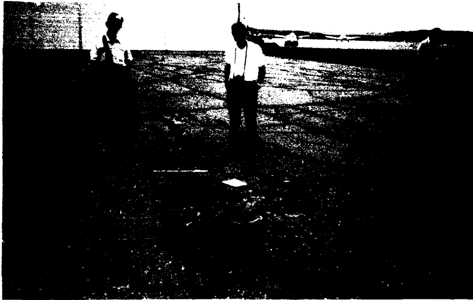
Figure 43. Disintegration in an AC parking apron.
