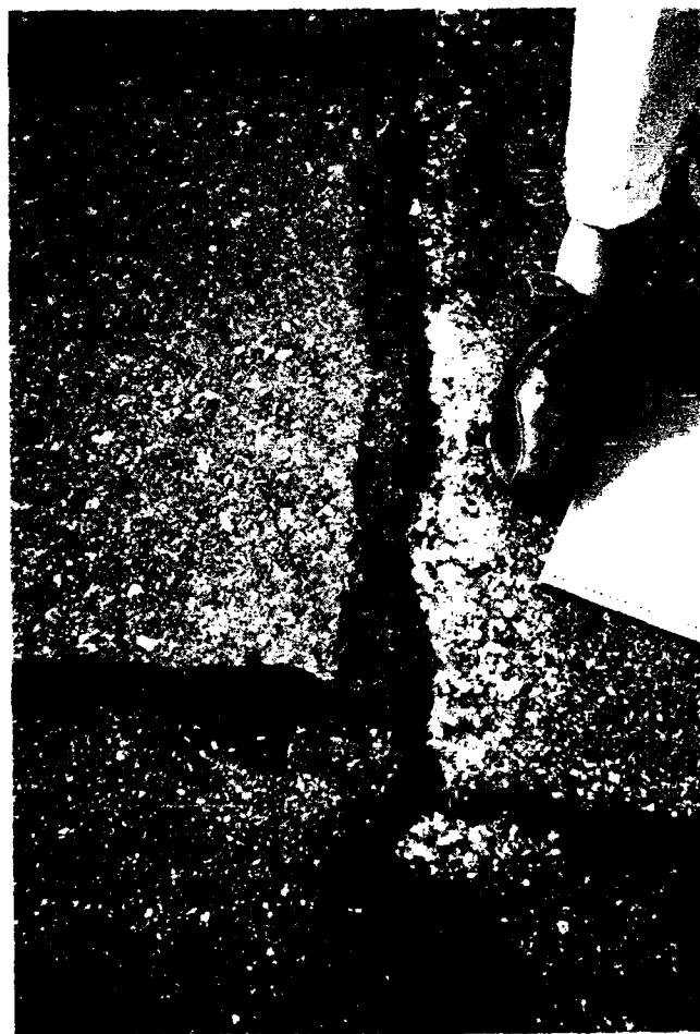
Figure 34. Distortion of AC pavement surface caused by frost heave.
