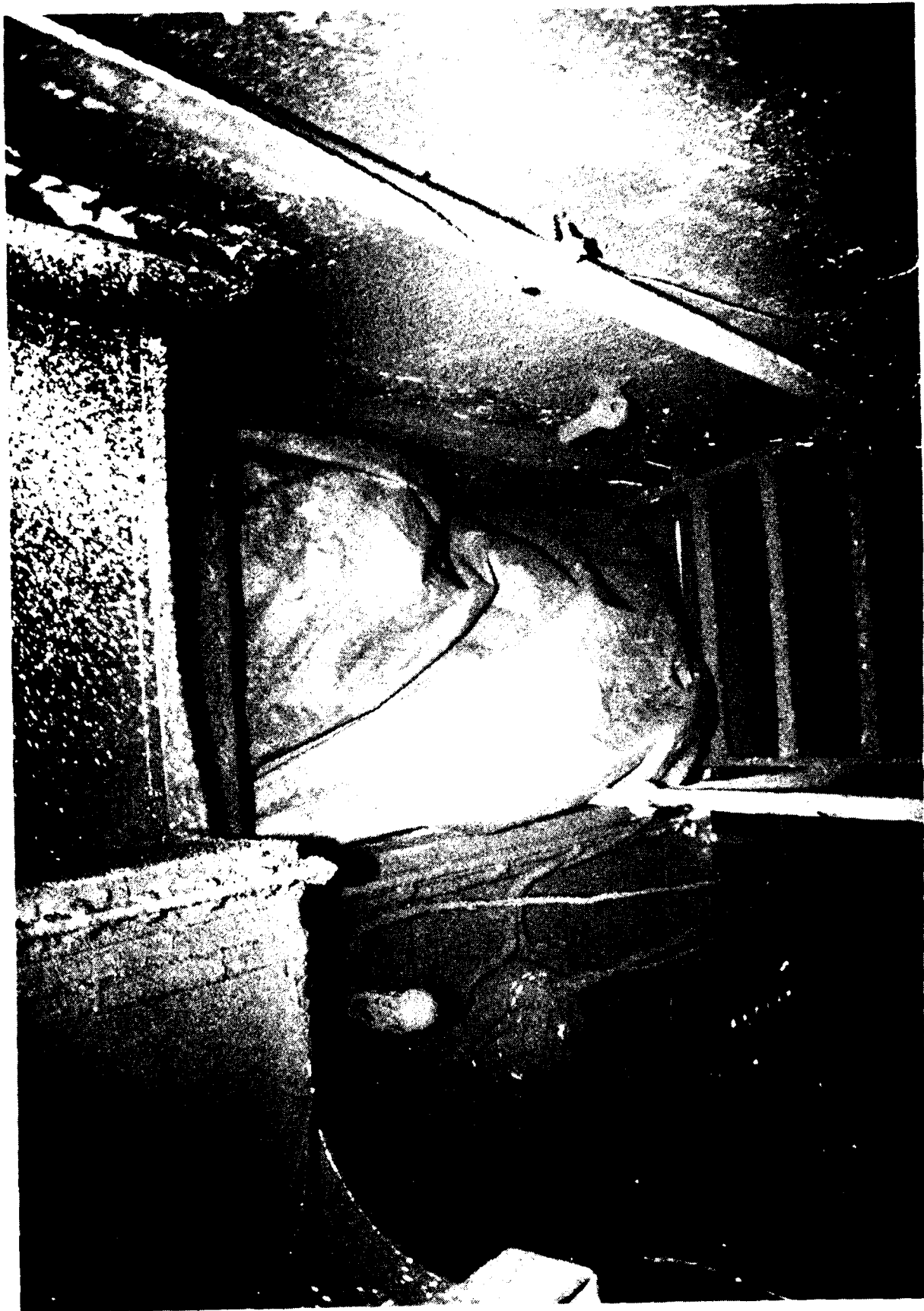
Fig. D-19 01 level thwart ships passage way - The smoke curtain in another test was deployed similar to D-18 photo.
