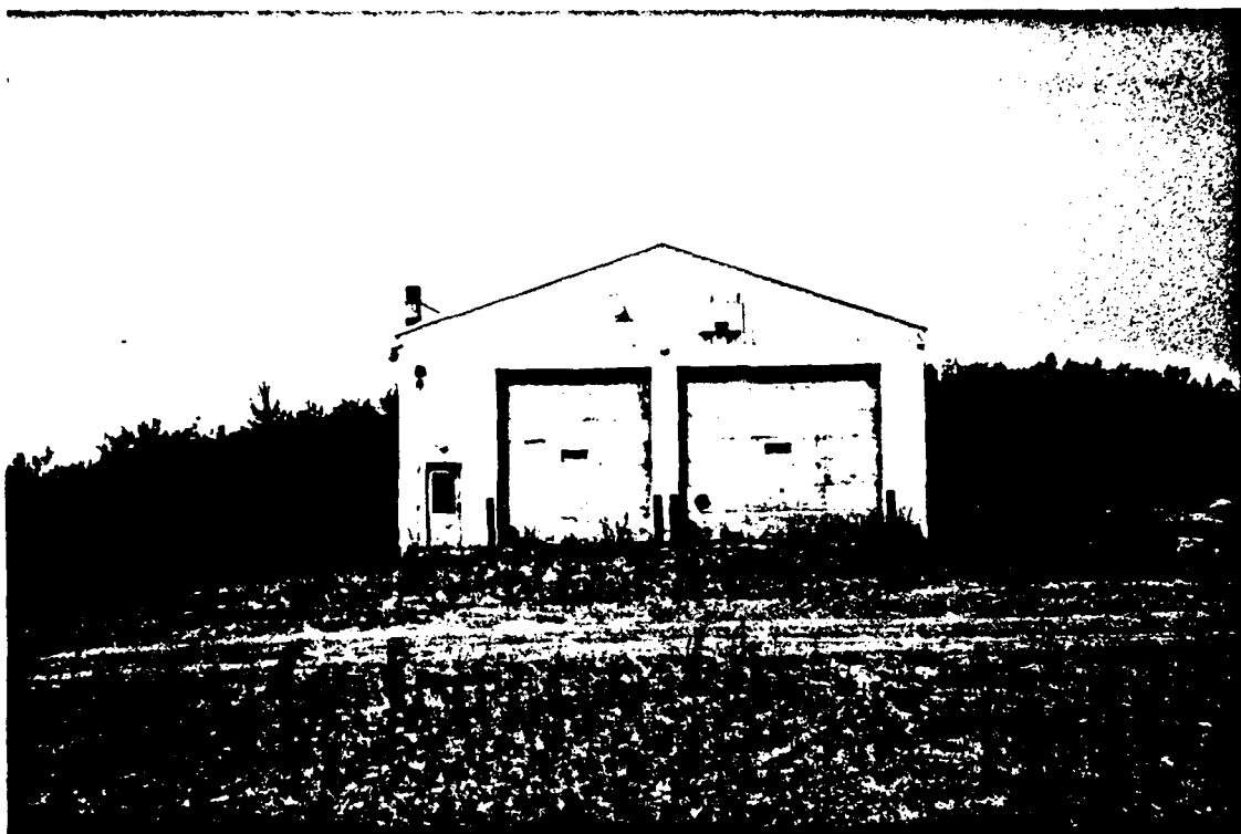
Photo 1. Vehicle maintenance shop at Bear Creek RRS.
