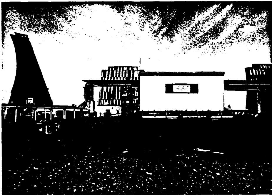
Photo 1. Bethel RRS-View Looking North, from left to right: Antenna No. 1, Facility Support Bldg., (front), Antenna No. 6 (back), Equipment Bldg, and Antenna No. 5.
