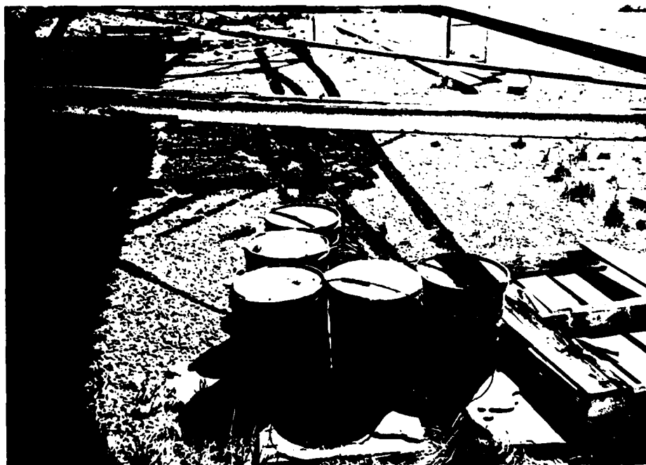
Photo 16. Site No. 3 - 5-Gallon Cans under Antenna No. 1.
