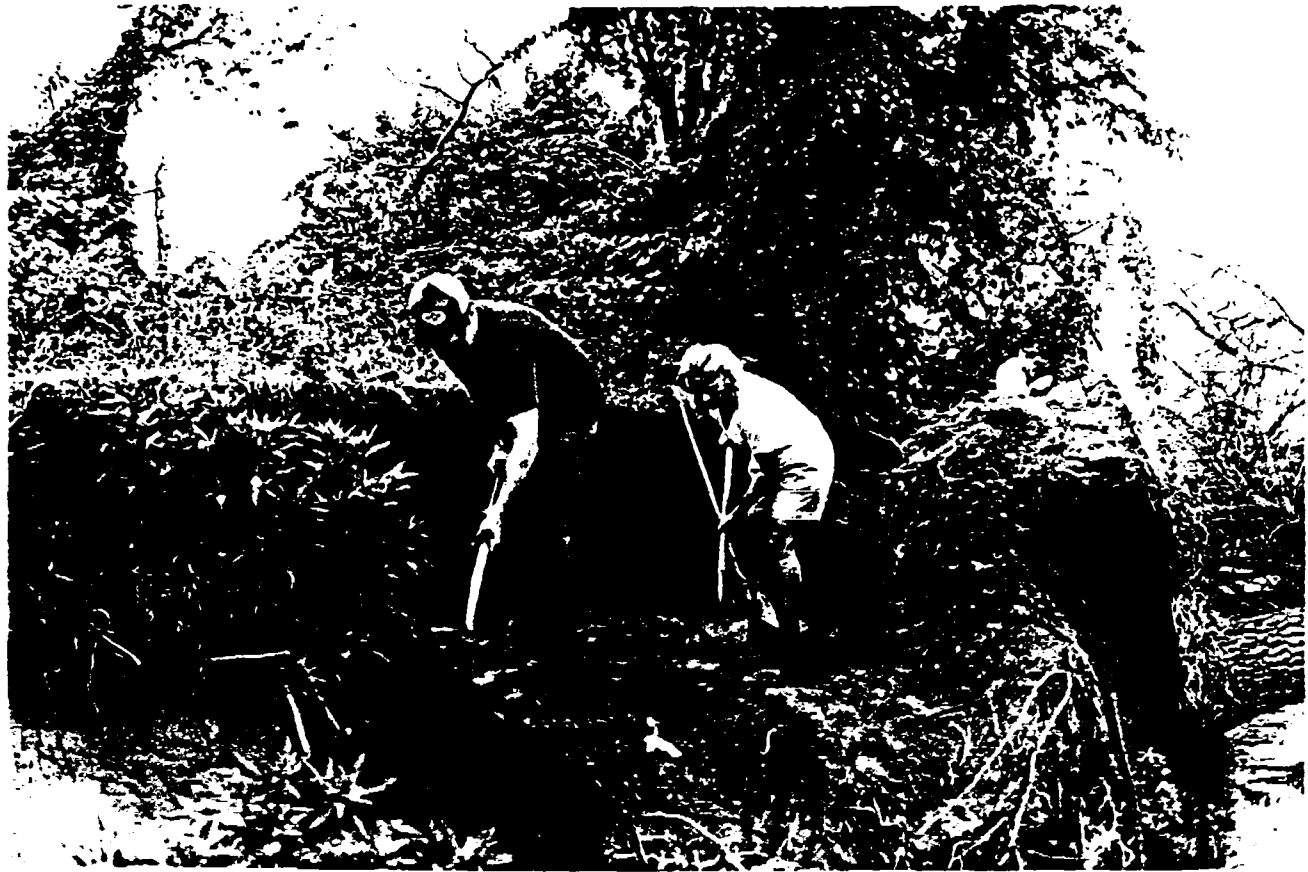
Figure 25: Skim shovelling bench beneath recently fallen red oak in 1987. Note grass platform to left, and root pull to right of excavators.
