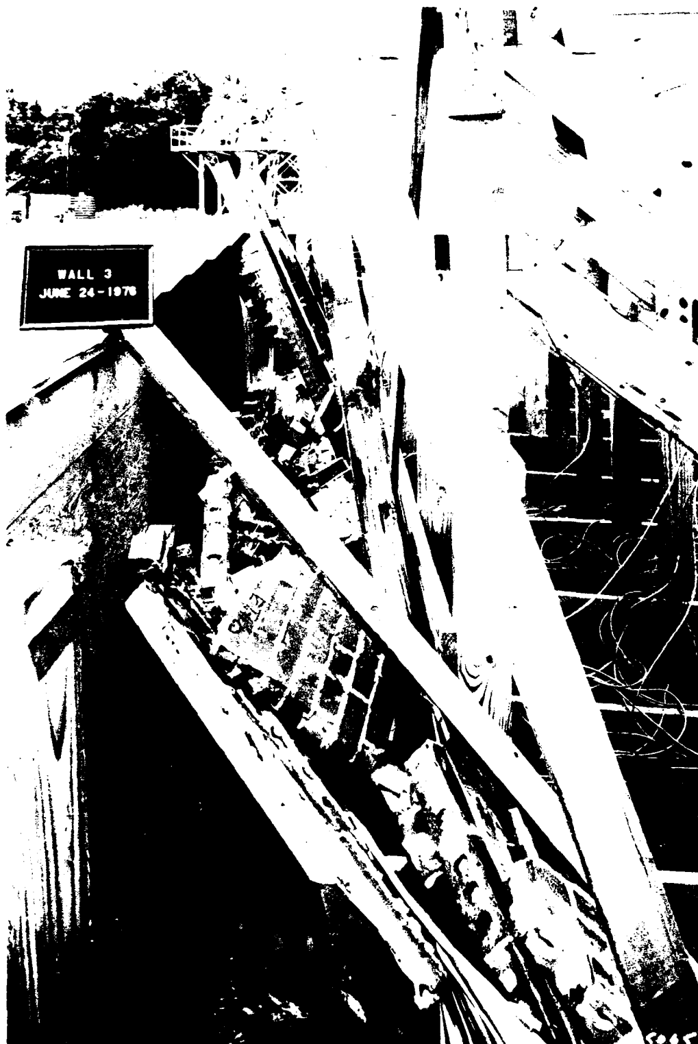
Figure 17. Wall 3. Wall failure, side view
