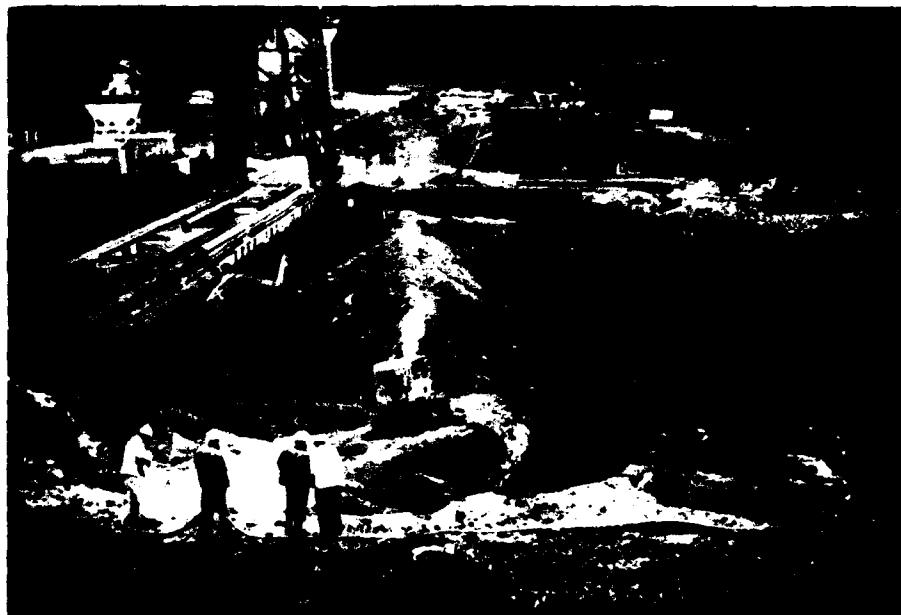
Right abutment, monoliths I-5 foundation cleanup with D-9 Cat, view east, 20 Oct. 1970.
