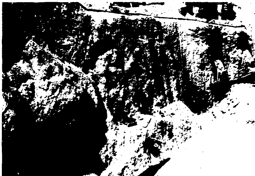
Mono. 6 cut slope with rock bolts and wire mesh on right canyon wall, view northwest showing workers preparing to blast lift between elevations 650 and 670 feet. Blast area is 35 to 100 feet downstream of dam axis, 10 Jul. 1970.
