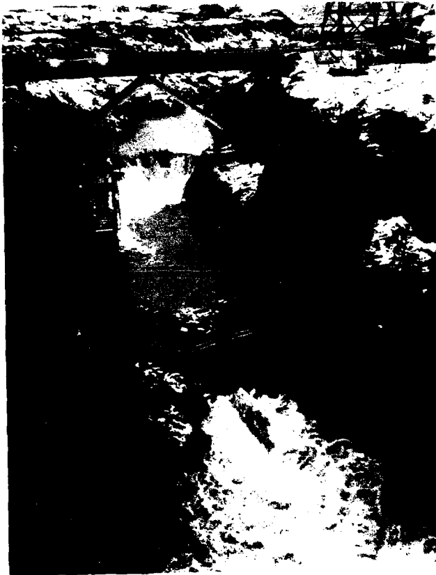
Completed coffer dam and diversion pipe, view upstream (north) showing flow overtopping at about 5200 c.f.s., 7 Dec. 1970.
