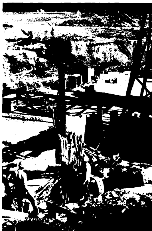
Monolith 12, view north showing Joy model 500 track drill boring "J" bar holes in foundation, 15 Sep. 1970.
