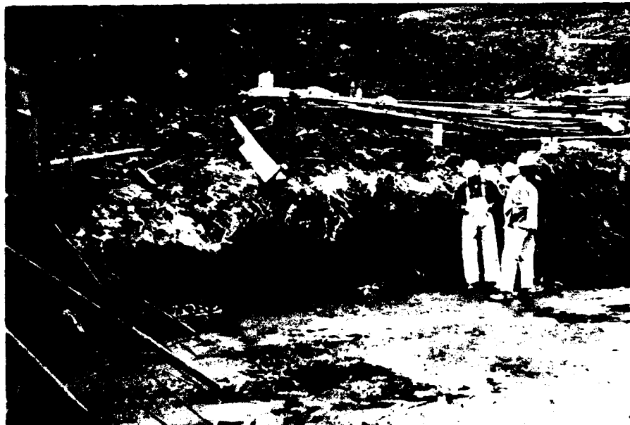
Mono. 1 foundation, view right (west) showing backfill concrete to elevation 750 feet, 9 Nov. 1970.
