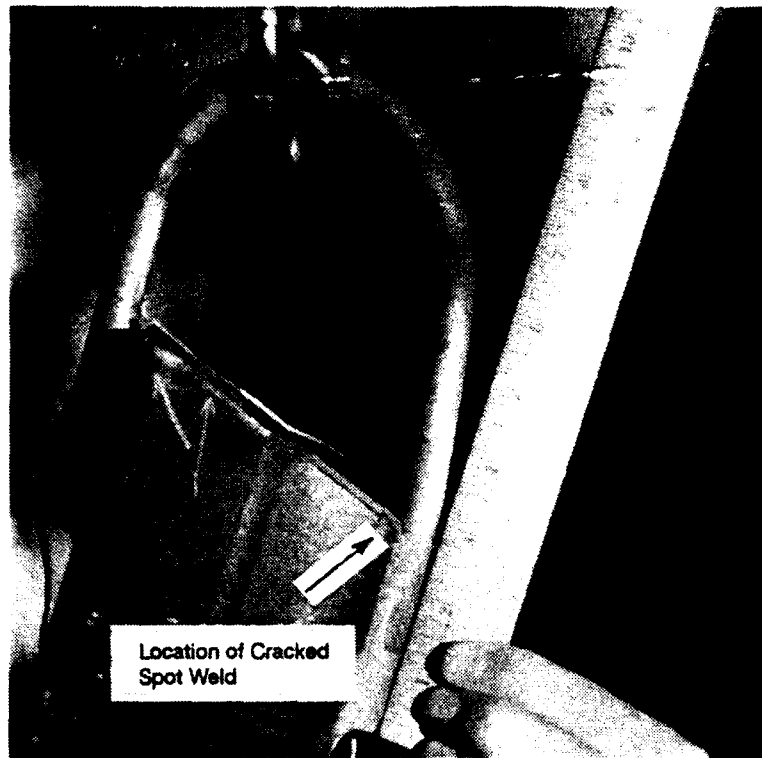
(a) Deformed provision and location of cracked spot weld
