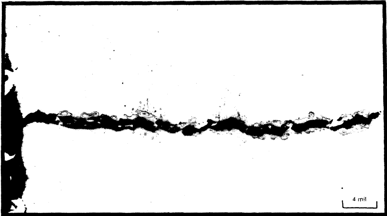
Figure 13. Crack in chain indentation sectioned transversely. Crack depth is approximately 0.040 in.
