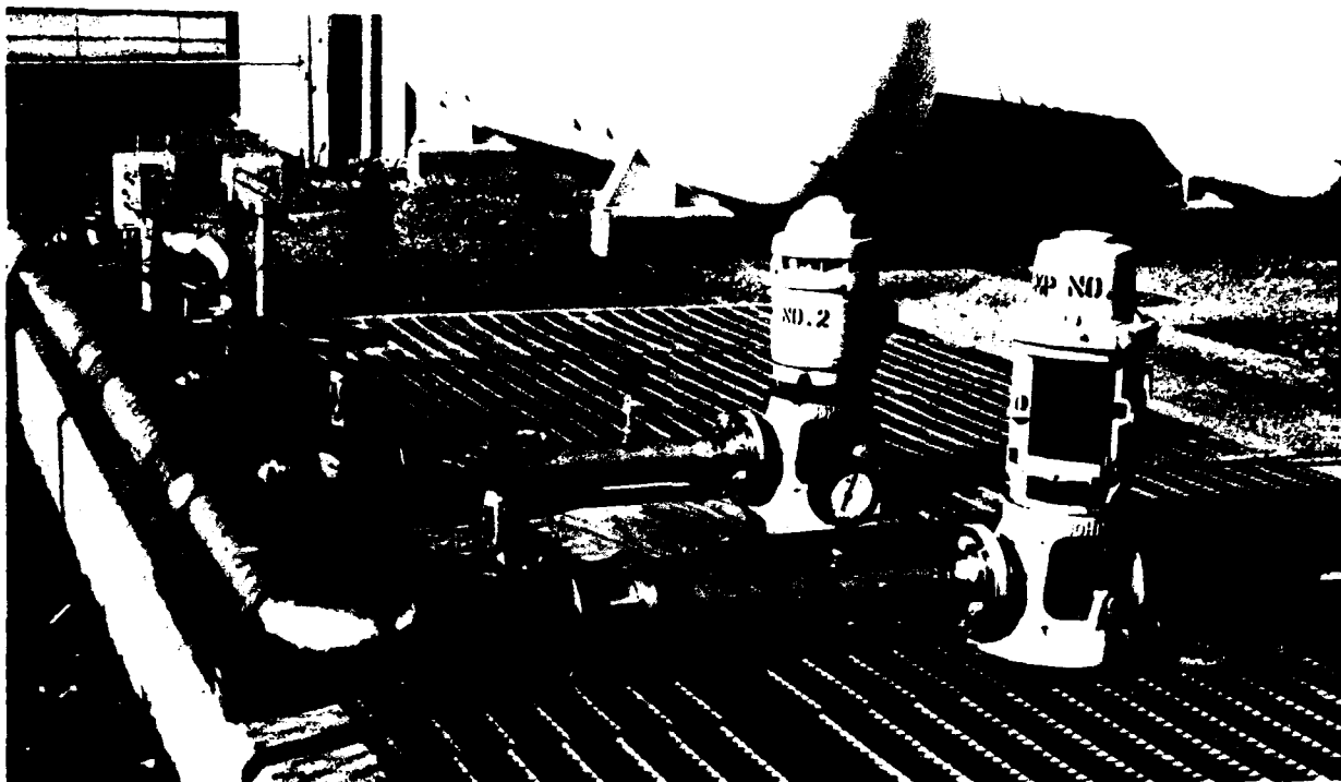
Figure 6. 9 RTS Precision Photo Lab Wet Well
