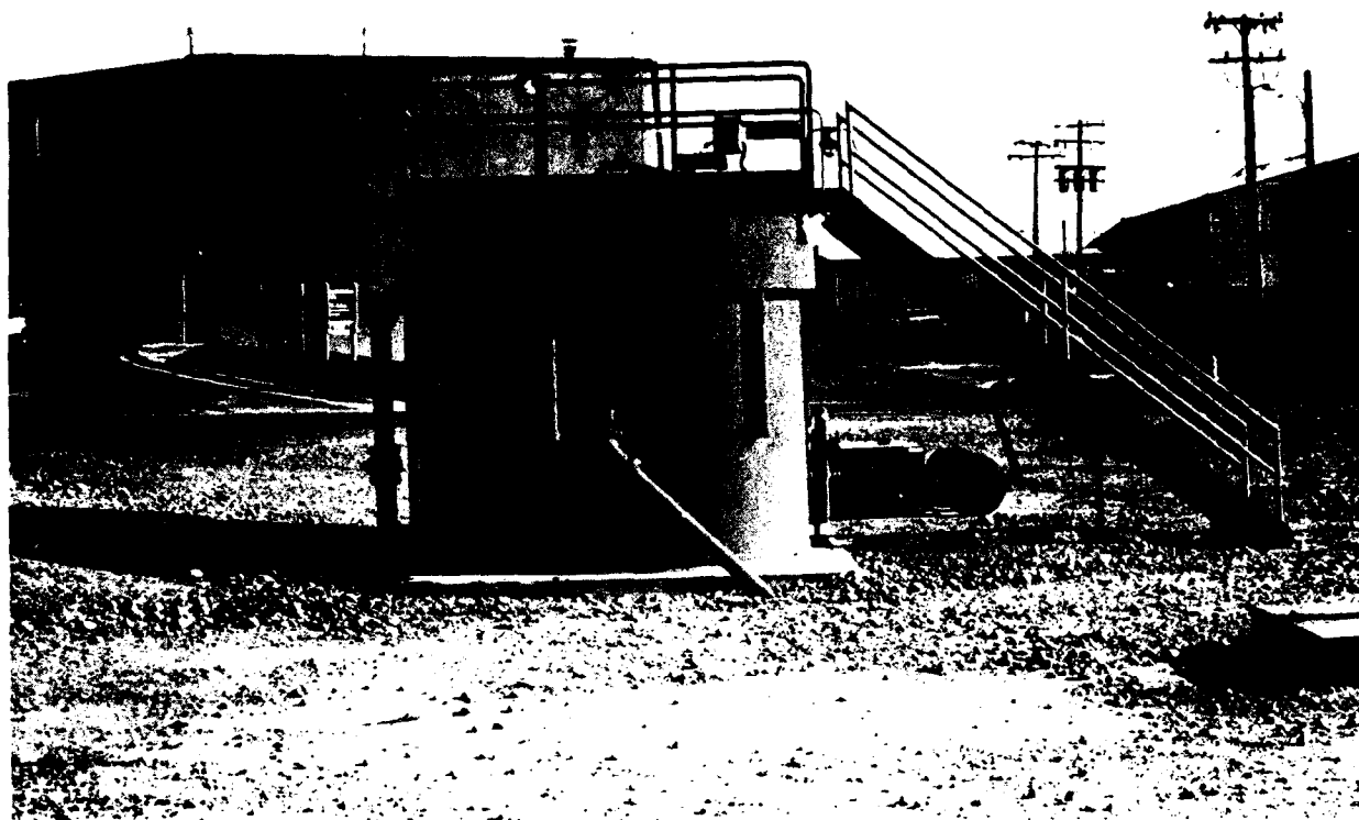
Figure 9. Washrack Oil/Water Separator
