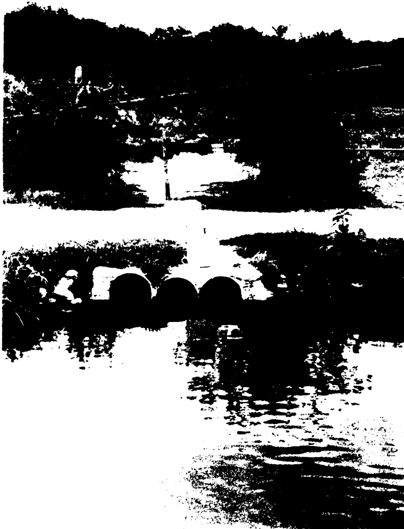
Figure 2: Effluent From Sewage Lagoon 2
