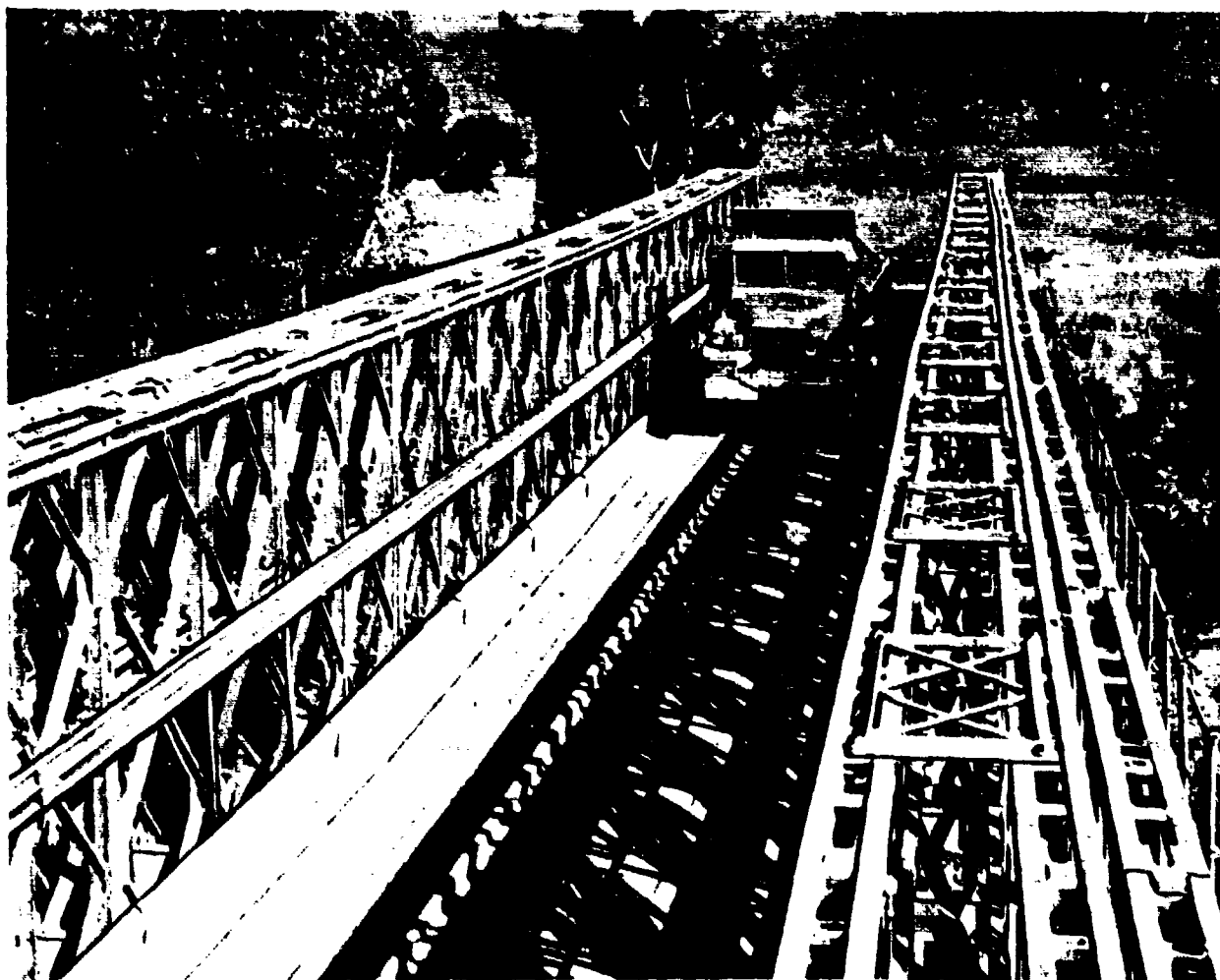
Figure 52. Example of a triple-truss double-story Bailey Bridge
