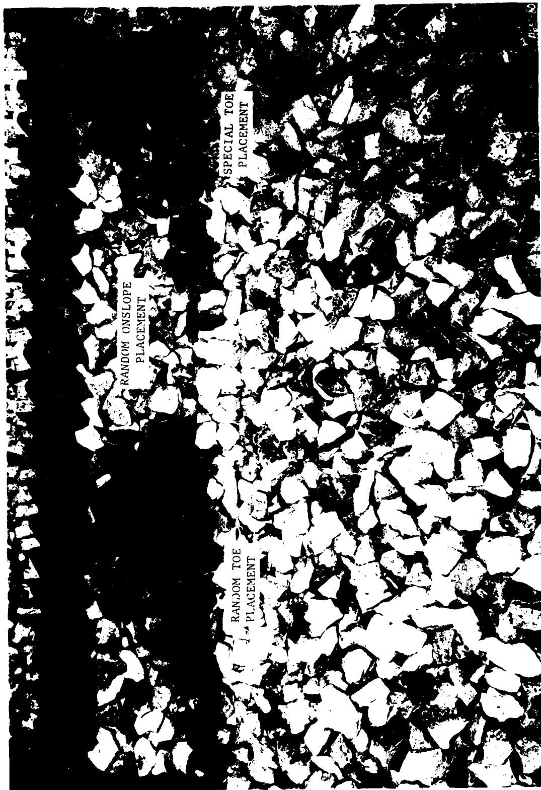
Photo A1. Comparison of random and special dolos toe construction.
