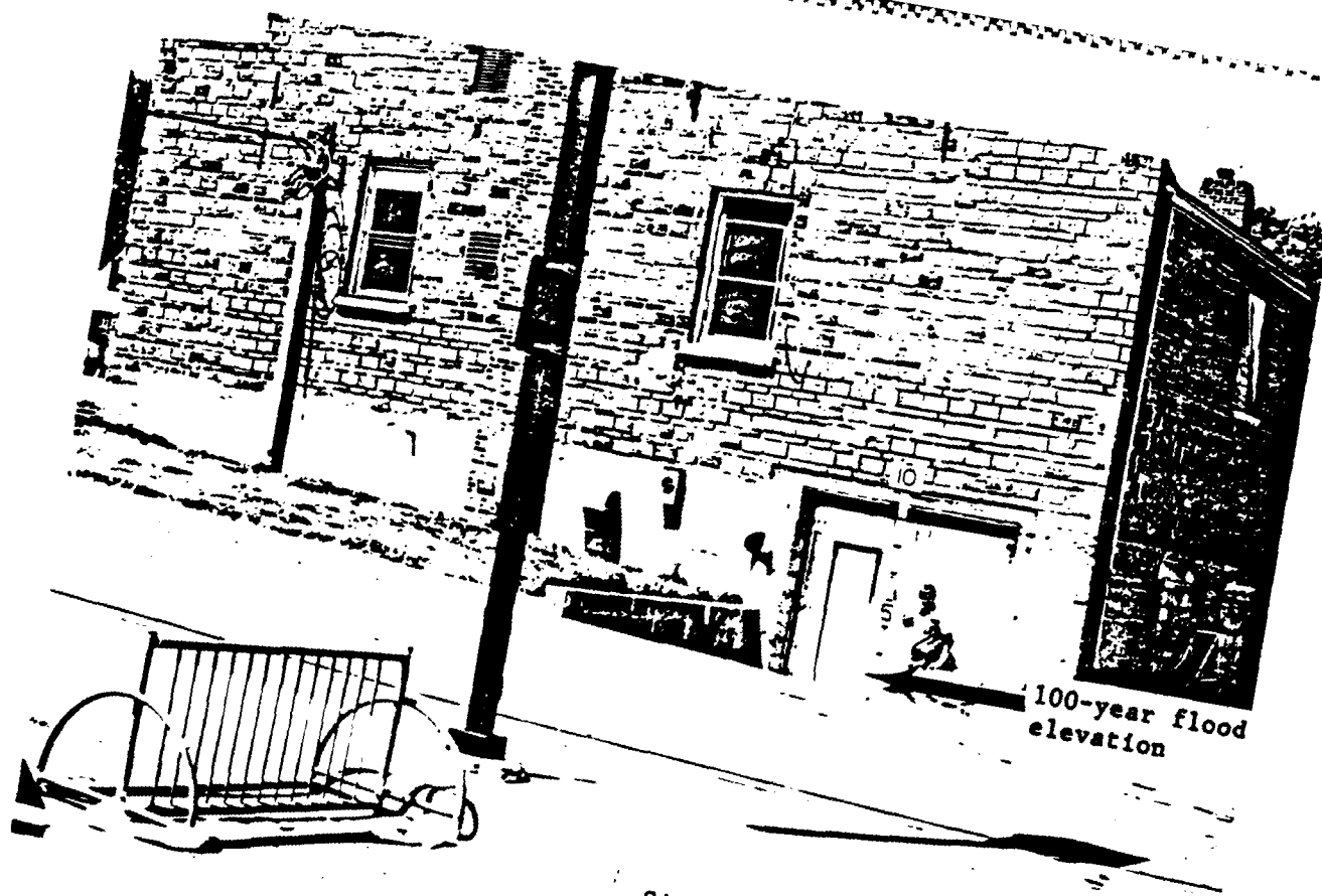
Site 16 Rear, August 85, Watertown, MN Note stoplog grooves PHOTOGRAPH 19
