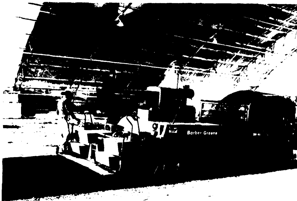
Photo 14. Placing of AC surfacing
