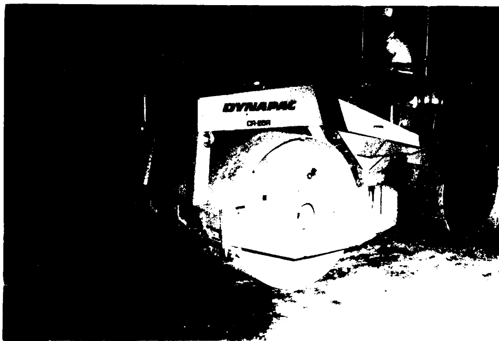
Photo 8. Vibratory roller used in compacting test section
