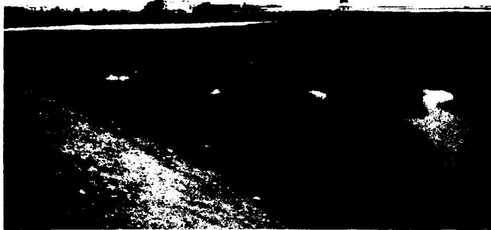
Figure 29. Roadside environment along the Prudhoe Bay Spine Road. Note the barren area caused by dust and water-filled ice-wedge polygon troughs. High-centered polygons have formed since the road was built in the 1970s. (Photo by D.A. Walker, 16 Aug 1983.)
