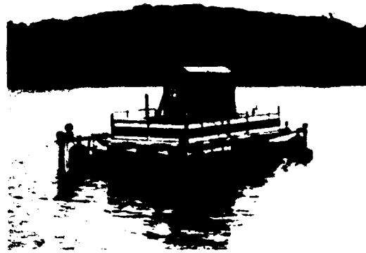
Figure 15. Oxygen Barge and Mooring Facility
