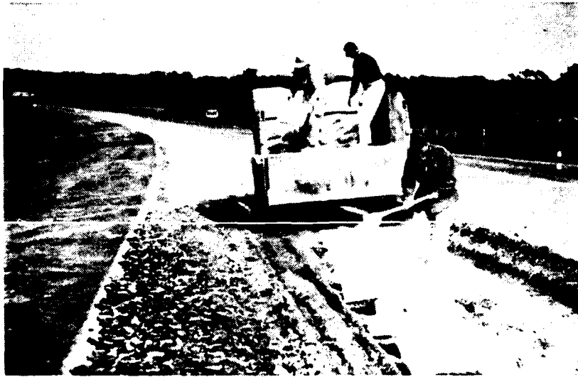
Figure 59. Bagged Lime Application.
