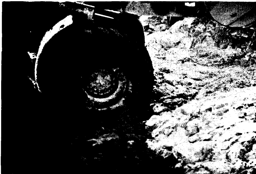
Photo 43. Front end loader with loaded bucket wheel rolling core material at rock-core contact. February 1984
