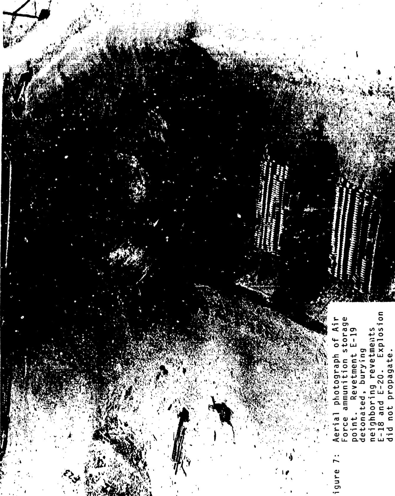
Figure 7: Aerial photograph of Air Force ammunition storage point. Revetment E-19 detonated, burying neighboring revetments E-18 and E-20. Explosion did not propagate.
