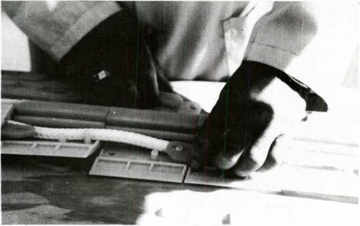
Figure 11. Installation of foreshortened 0.5-inch, double-braided nylon safety line within fairing.
