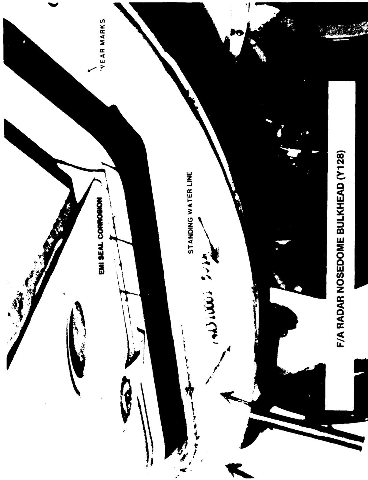
Figure 2 - Corrosion under the EMI-seal area in the F/A-18 Radar Nosedome Bulkhead (Y128).
