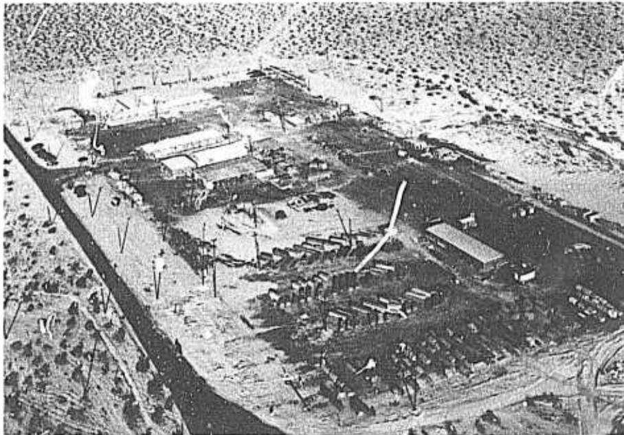
Salt Wells Pilot Plant under construction, July 1945.
