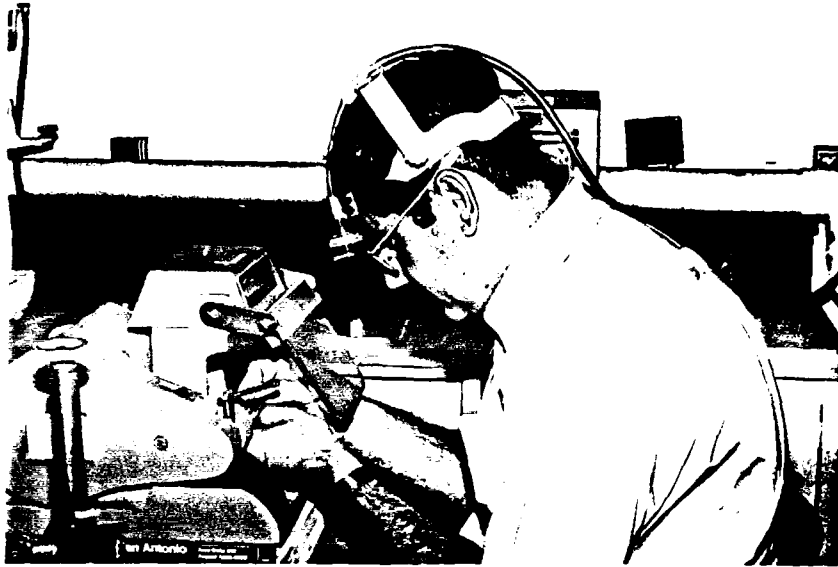
Figure 10. Technician wearing alpha-1 sample pump. (Note: filter is located in breathing zone of operator.)
